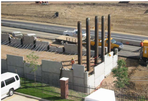
Figure 5. MSE construction at Dry Creek Rd
