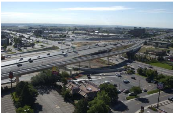
Figure 2. LRT Bridge over Arapahoe Rd
