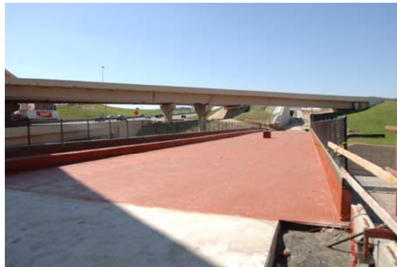
Figure.10. Spray applied waterproofing system of LRT over C-470.
