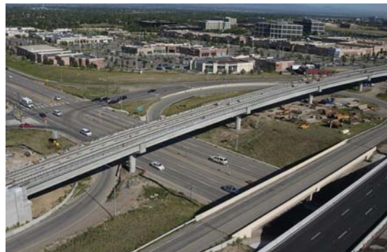
Figure 3. LRT Bridge over County Line Rd
