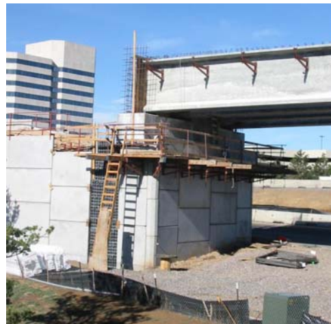
Figure 6. MSE construction at Orchard Rd
