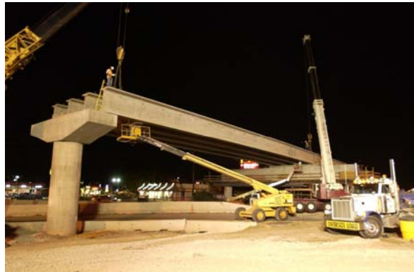
Figure 4. Girder Erection at Arapahoe Road
