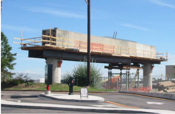
Figure 13. CIP straddle bent construction
