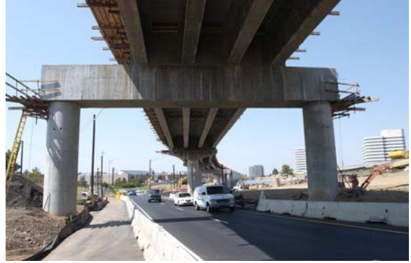
Figure 14. CIP straddle bent construction
