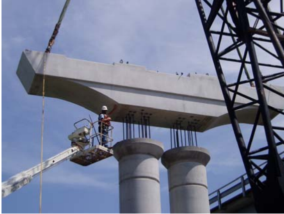
(a) Lake Belton Bridge, TX (14)
