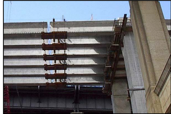
Photo 3. Strongbacks Supporting Span Segments
