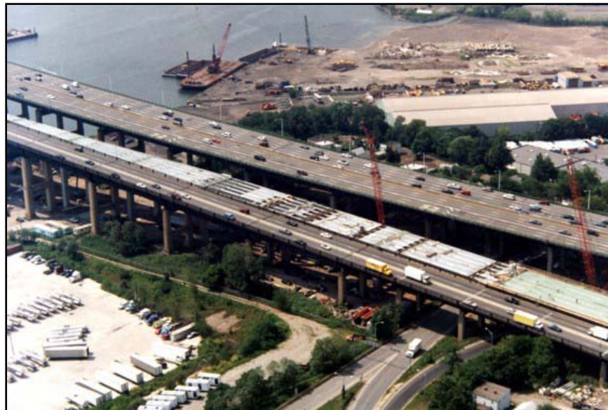
Photo 9. Construction at North End (Looking South West)
