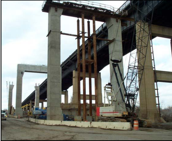
Photo 2. Temporary Girder Support at Pier
