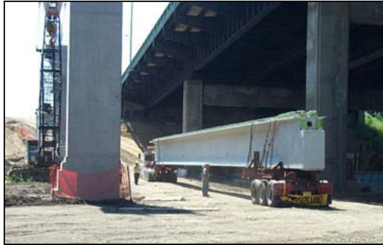
Photo 4. Delivery of Girder
