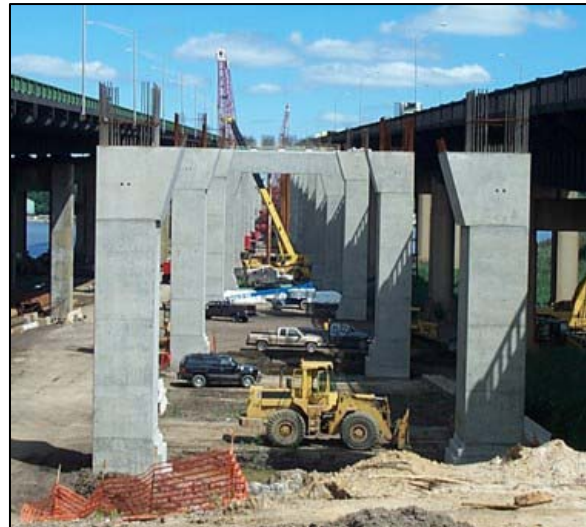
Photo 5. Pier Construction Looking North
