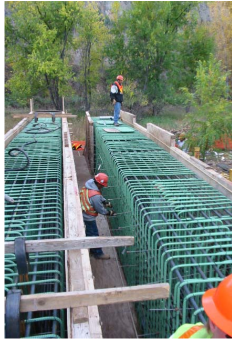
Figure 8. Fabricating the pier caps
