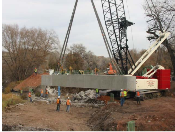
Figure 9. Precast pier cap installation
