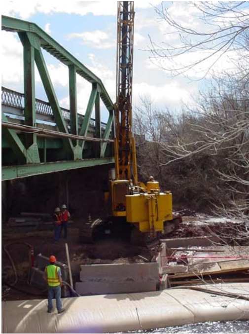
Figure 7. Pier caisson construction
