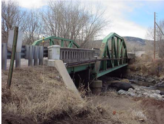
Figure1. One of two existing structures
