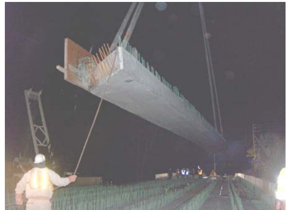
Figure 11. Girder erection
