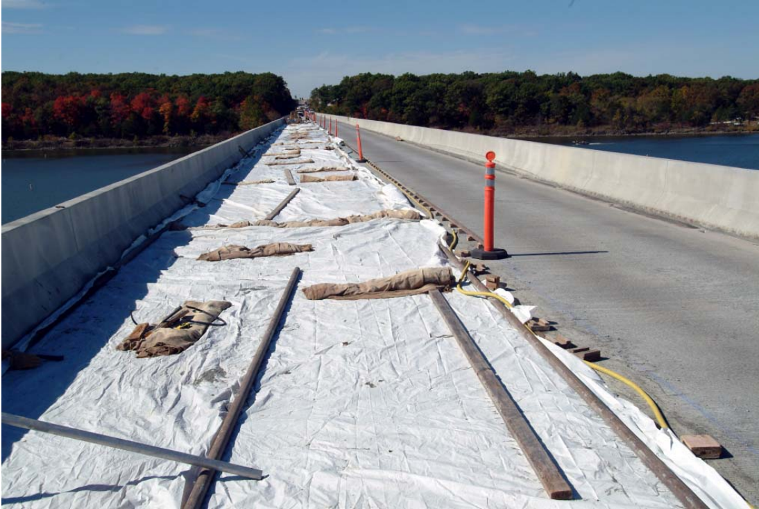
Figure 5. Stage Construction at End of Project
