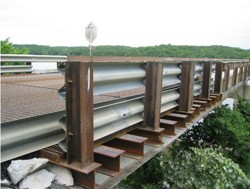
Figure 4. Temporary Deck Panel
