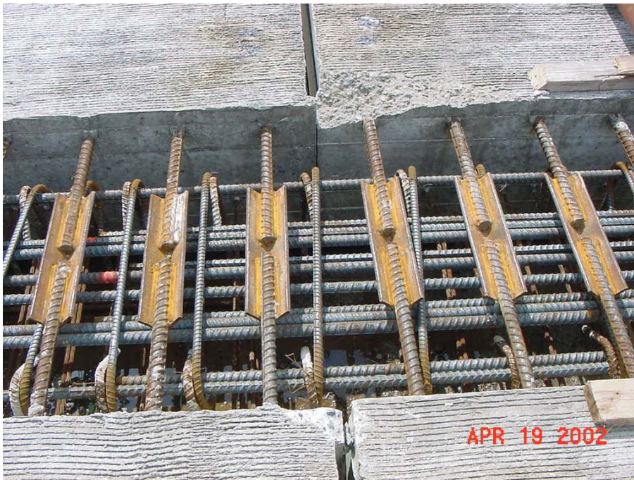
Figure 13: Photograph of Deck Panel Top Bar Connection
