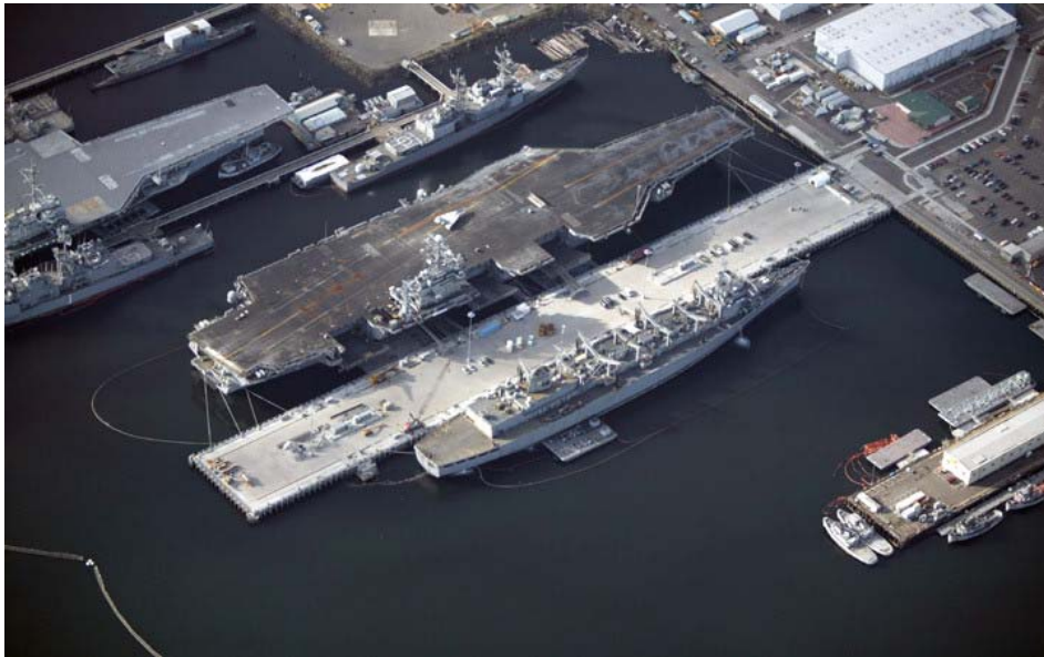
Figure 1: Completed Pier Delta
