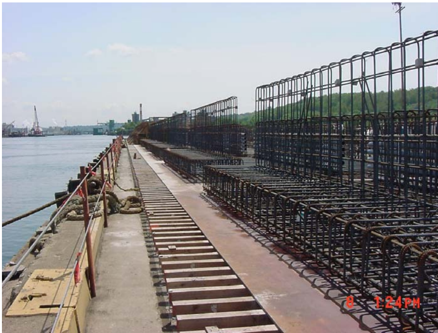
Figure 14: Site Precasting of Utilidors
