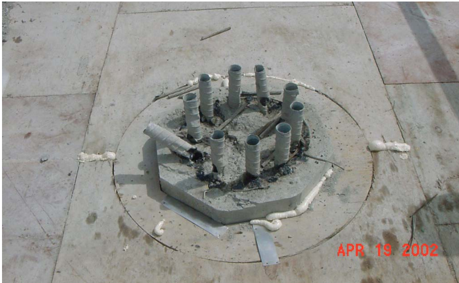
Figure 11: Photograph of Typical Pile Connection with Dowels
