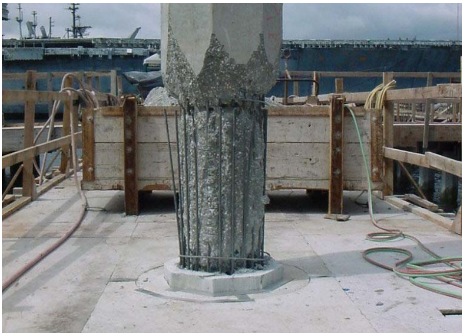
Figure 12: Photograph of Alternate Pile Connection with Strand
