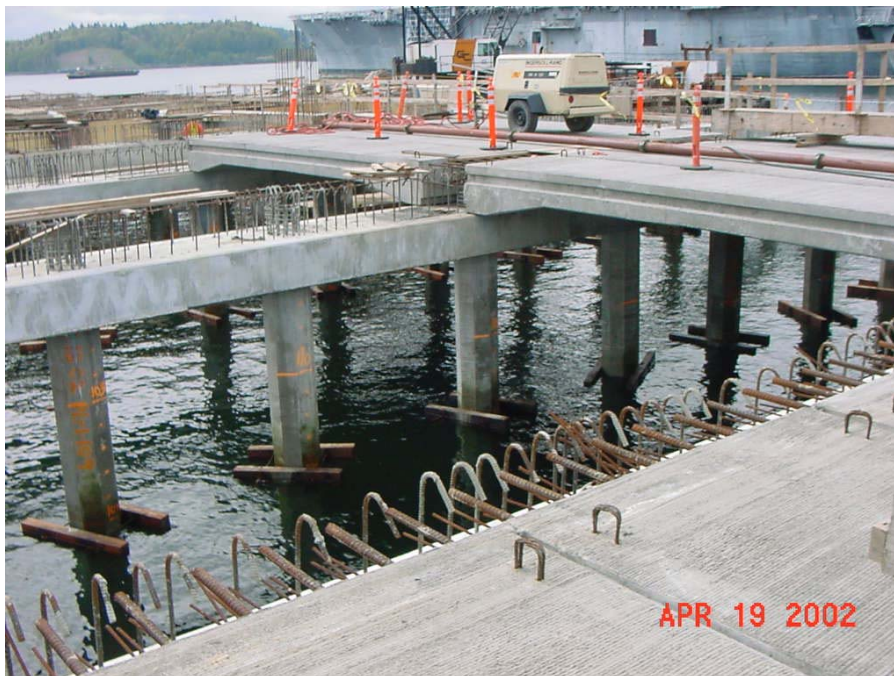
Figure 3: View of Deck Panels, Pile Caps, and Piles under Construction
