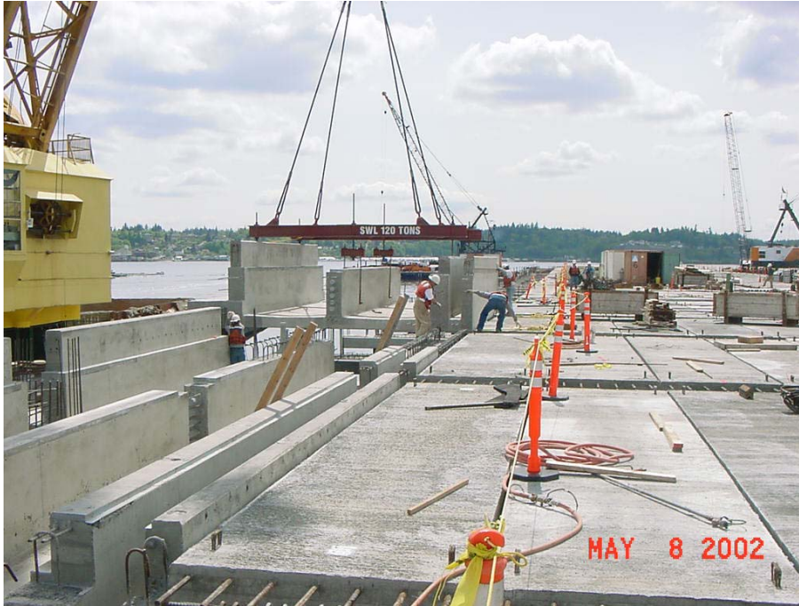
Figure 4: View of Precast Concrete Utility Tunnel Being Erected
