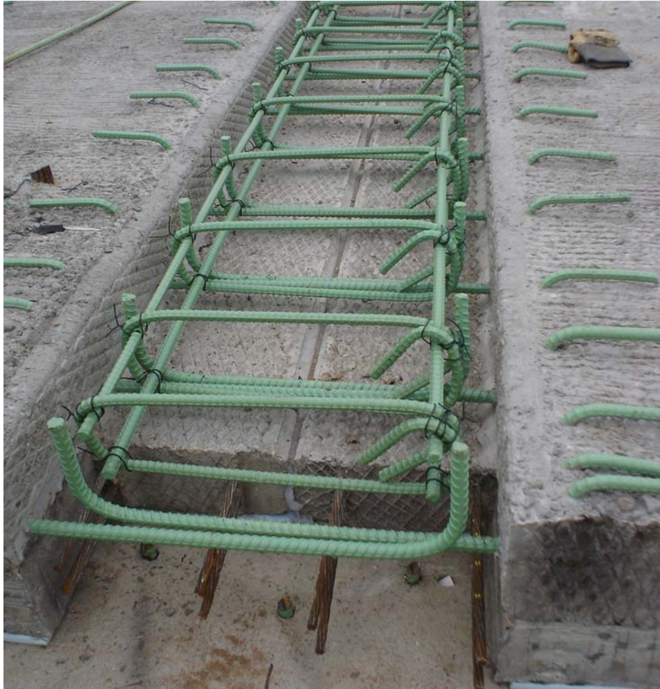
Figure 5. Drop-In Reinforcement at Construction – Center City Bridge.
