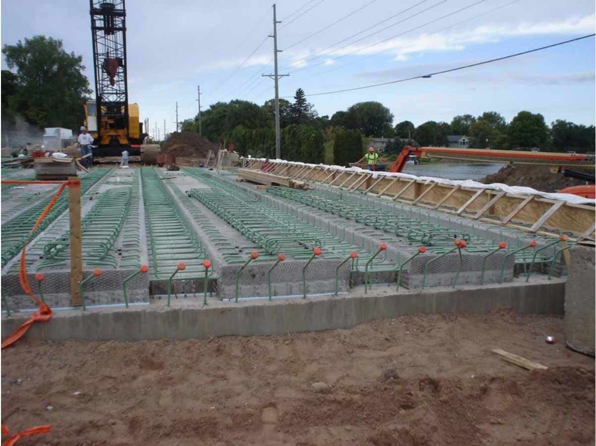
Figure 11. Stage 1 Construction – Center City Bridge.
