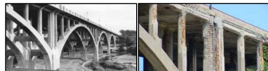
Fig. 1 Existing Fulton Road Bridge (1932 and Today)
