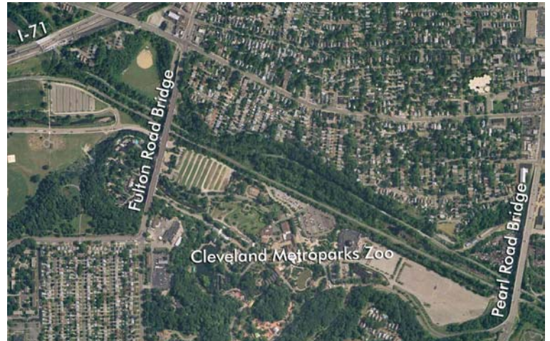
Fig. 2 Fulton Road Bridge Site
