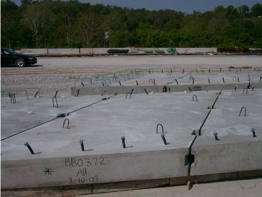
Figure 6 - Panels in the Yard – Mock-up Test
