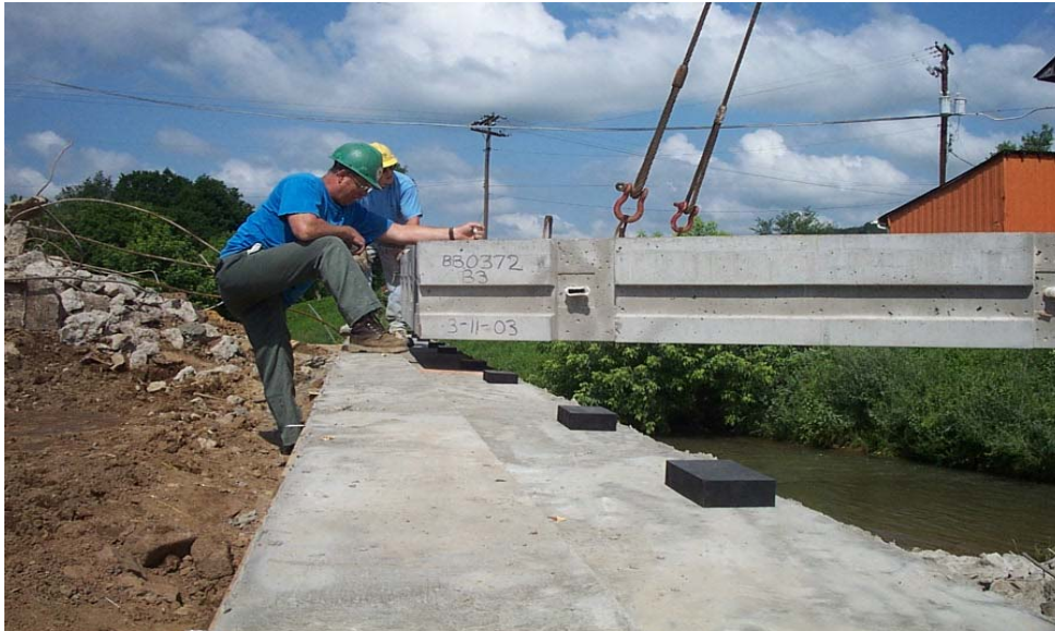
Figure 7 - Placing the Deck Slabs, Transverse PT Ducts are Visible
