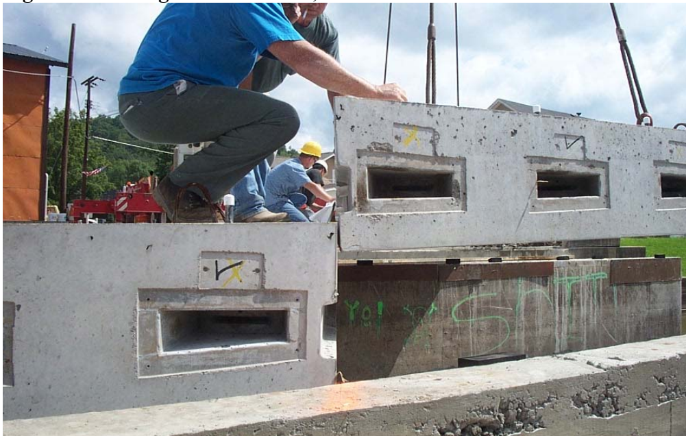
Figure 8 - Slab Placement - Longitudinal PT Ducts Are Visible
