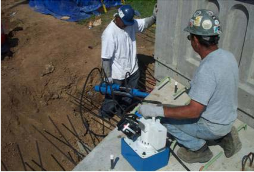
Figure 11 – Post-tensioning
