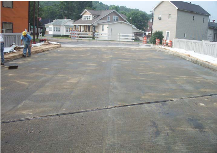
Figure 12 – The Completed Bridge
