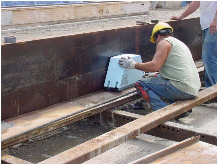
Fig. 7 Blockouts for top strand beams
