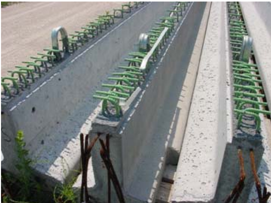
Fig. 1 “Bug” holes in bottom flange of IT
