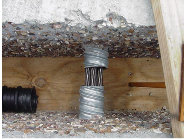
Fig. 12 Exposed aggregate roughened surface used in the Arch Tied Bridges, Texas
