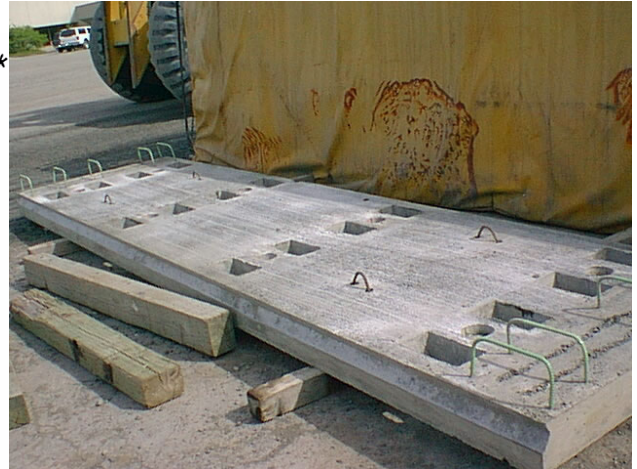
Fig. 13 Non-reinforced panel-to-panel connection used on bridges by ADOT
