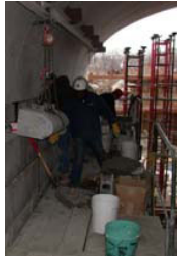
Figure 6 Setting Cutwater Cap
