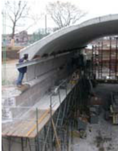
Figure 23 Pre-cast Arches and Rail
