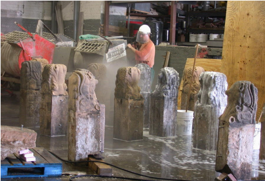
Figure 21 Cleaning the Animal Heads
