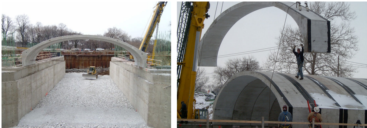
Figure 11 Arches under Construction
