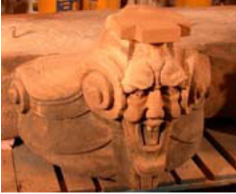
Figure 22 Mortar Patches
