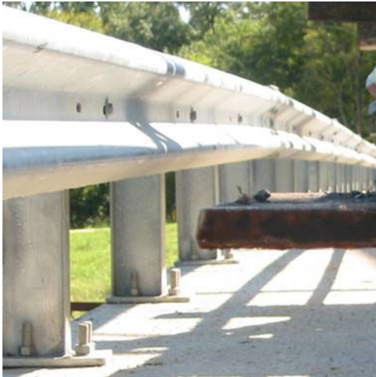
Fig. 13 Texas Type T6 Bridge Rail
