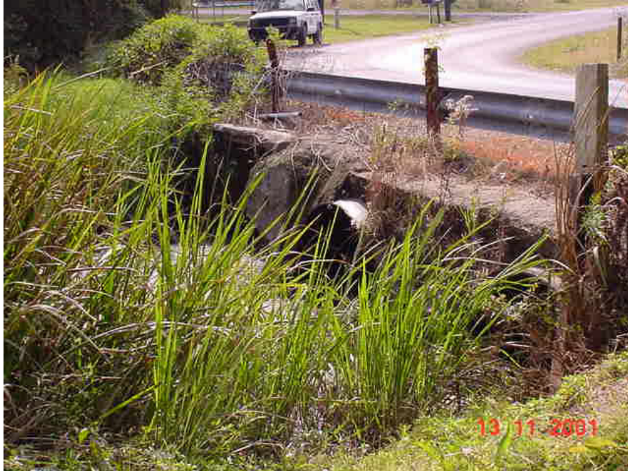
Fig. 2 Existing Structure to be Replaced.
