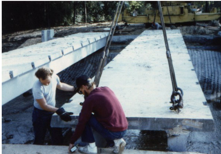
Figure 8. Double-Tee Bridge System
