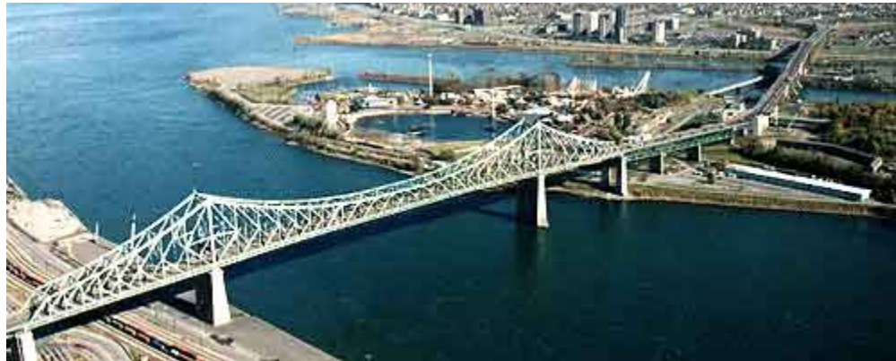
Figure 3. Jacques-Cartier Bridge (Source: www.pjcci.ca )
