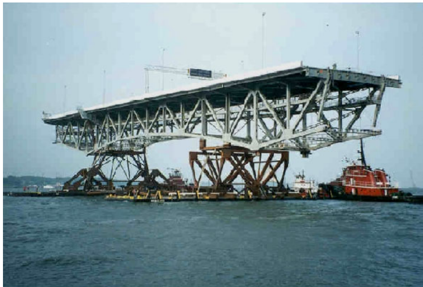
Figure 11. George P. Coleman Bridge (Photo Credits: Virginia Department of Transportation)
