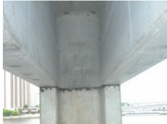
Figure 16. View of Prefabricated Substructure and Girders of Edison Bridge
