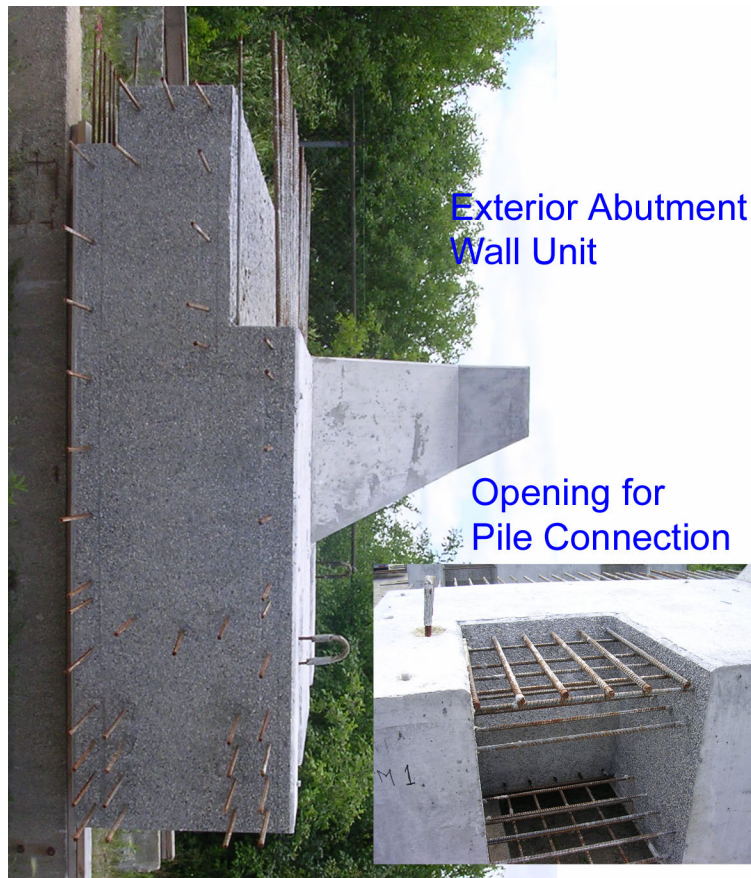
Fig. 10 Typical Exterior Abutment Wall Unit
