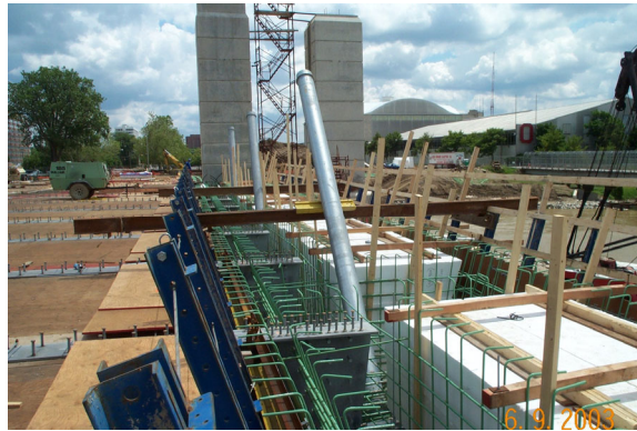
Fig. 16 View of cast-in-place edge girders
