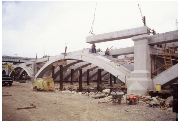
Fig. 5 Setting prestressed box beams on precast arch units and pier
