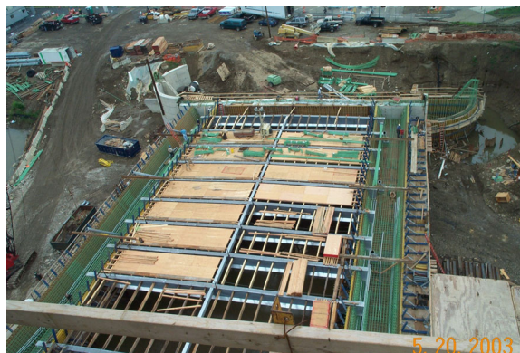
Fig. 17 Revised floor system with cast-in-place edge girders
