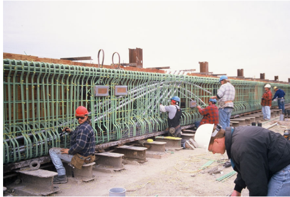
Fig. 8 Fabrication of precast edge girder section
