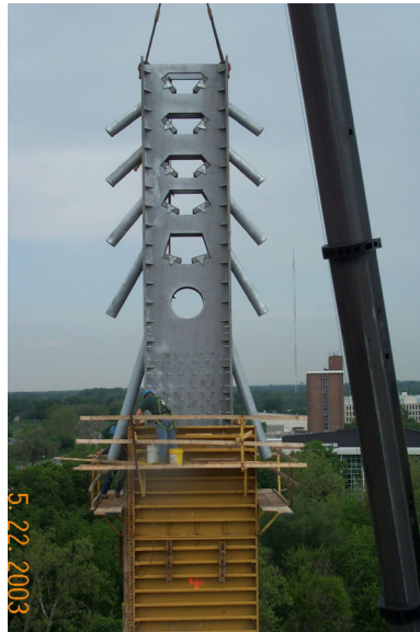
Fig. 18 View of the upper tower anchorage
