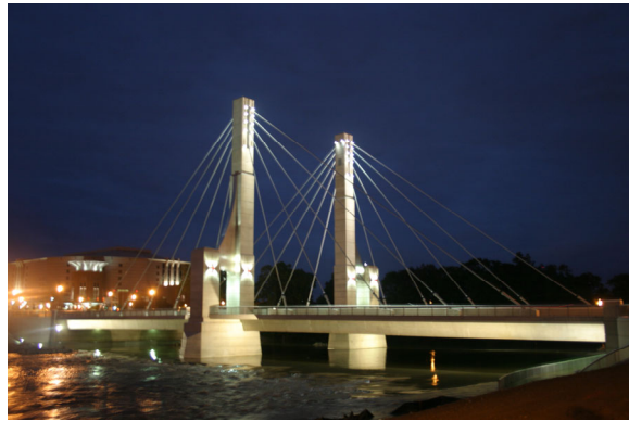
Fig. 15 Lane Avenue Bridge with architectural lighting
