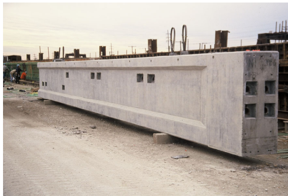
Fig. 9 Finished edge girder section
