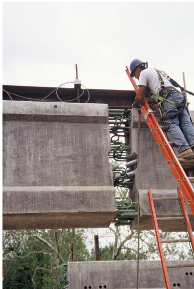
Fig. 7 Beach Road edge girder splice section
