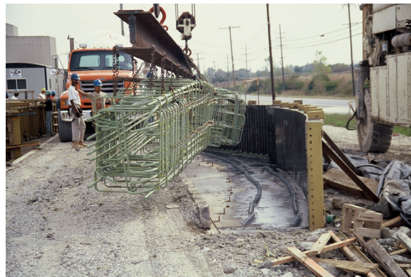
Fig. 4 Placement of reinforcing steel cage for arch rib section
