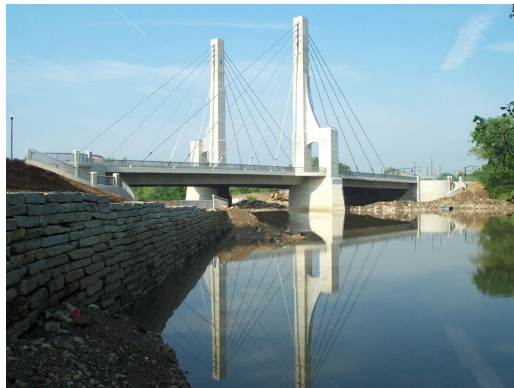
Fig. 19 Completed Lane Avenue Bridge
