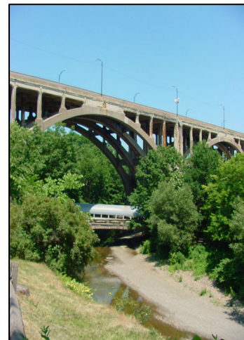
Brookside Park Bridge and Big Creek Under Fulton Road Bridge
