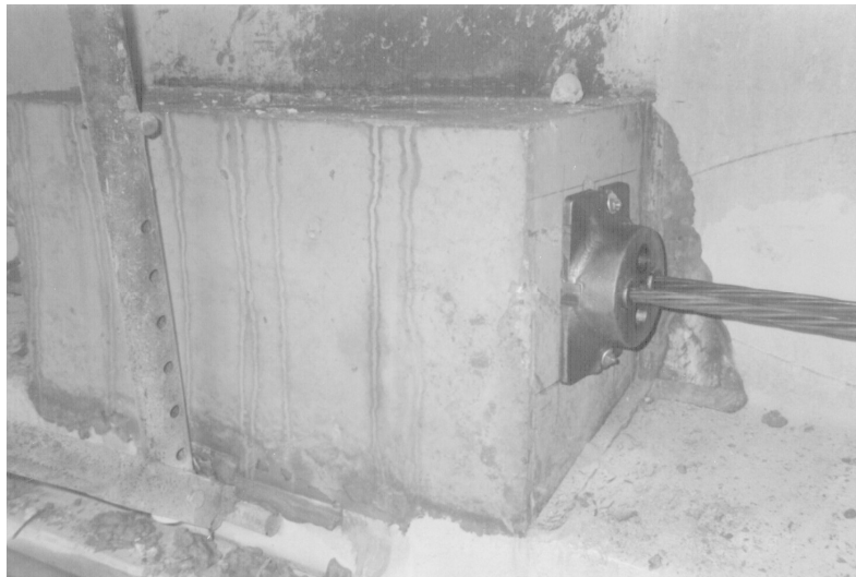
Anchor Block with Post-tensioning Strands
