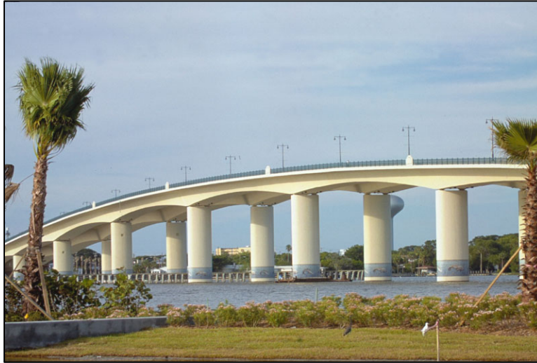
Figure 5 – Broadway Bridge: Recipient of 8 major design awards for FDOT.
