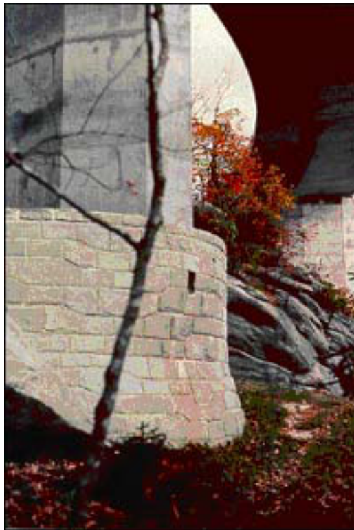
Figure 3: Linn Cove Viaduct: Concrete mix designed to blend with the mountain.
