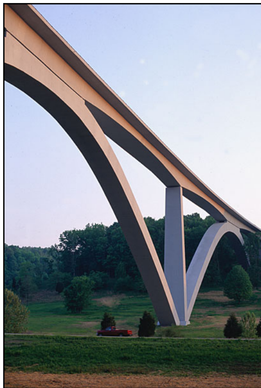
Figure 4 – Natchez Trace Parkway Arches: First precast segmental arch in the U.S.
