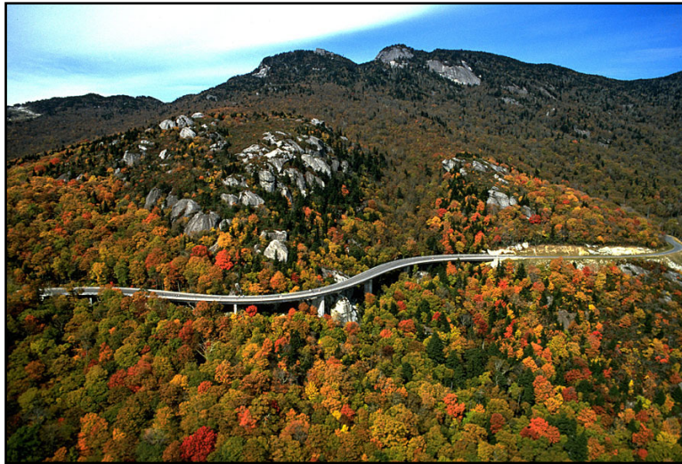
Figure 2: Linn Cove Viaduct: Built from the top to protect the environment.
