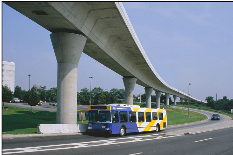
Figure 7 – JFK Light Rail System: Concrete mix designed for uniform concrete color.
