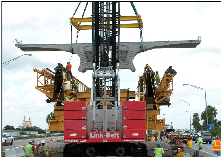
Figure 8 – Lee Roy Selmon Crosstown Expressway: Under construction, showing unique sculpted superstructure shape.
