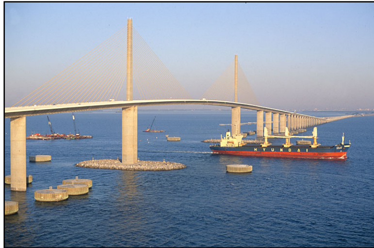
Figure 1: Sunshine Skyway Bridge: Icon for Tampa/St. Petersburg, Florida.
