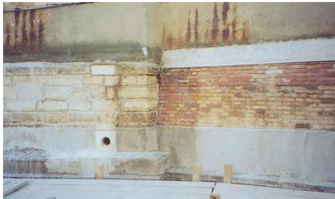
Fig. 26 400-year-old Structure Restoration, Venice, Italy 2002
