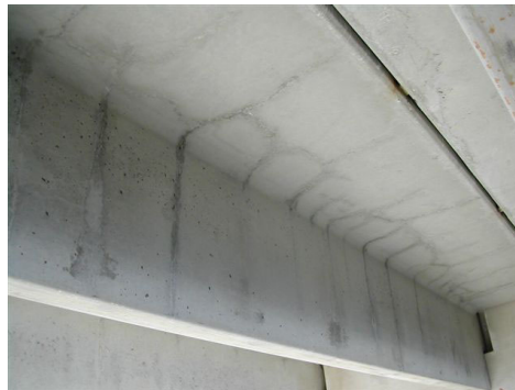
Fig. 2 Underside Parking Deck – Precast Tees
