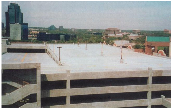
Fig. 9 Northside Hospital, Atlanta, Georgia, 1999
