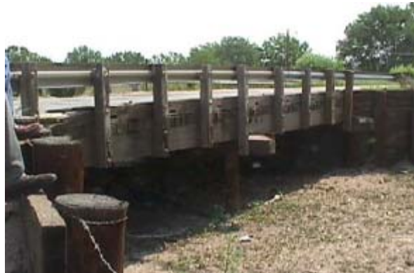
Fig. 1 Mitchell Gulch Bridge before Replacement
