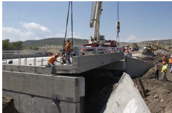
Fig 4 Outside Girder with Curb and Railing
