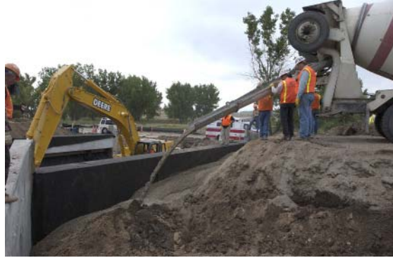
Fig 3 Both Abutments in Place
