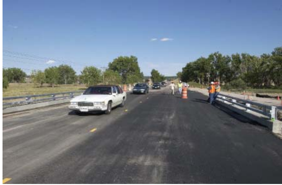
Fig 5 New Mitchell Gulch Bridge Open to Traffic
