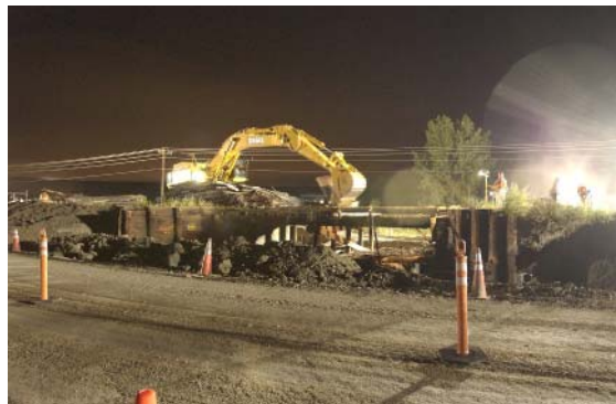
Fig. 2 Demolition of the Old Mitchell Gulch Bridge
