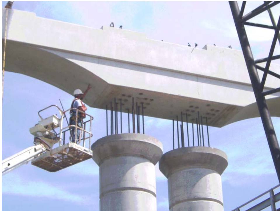
Setting a precast cap onto the connection dowel
