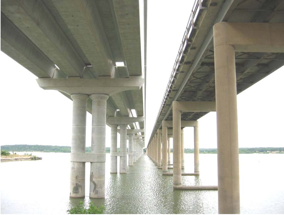
Partially completed Phase 1 on left, existing bridge on right.
