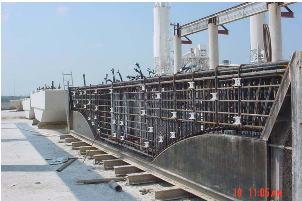
Formwork, reinforcing and completed caps in casting yard
