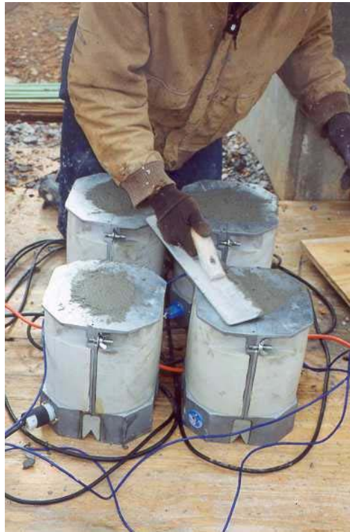
Fig. 1 Preparation of match-curing concrete batch material samples
