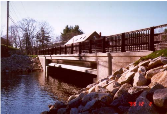
Figure 1 ~ Bristol 2 - 2000 PCI Award Best Bridge Span less than 65'
