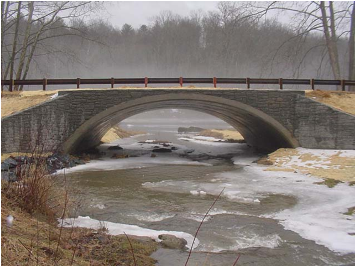
Figure 4: The stone arch look of the completed project was achieved by using concrete form liners. Due to low temperatures, the concrete stain has not yet been applied.
