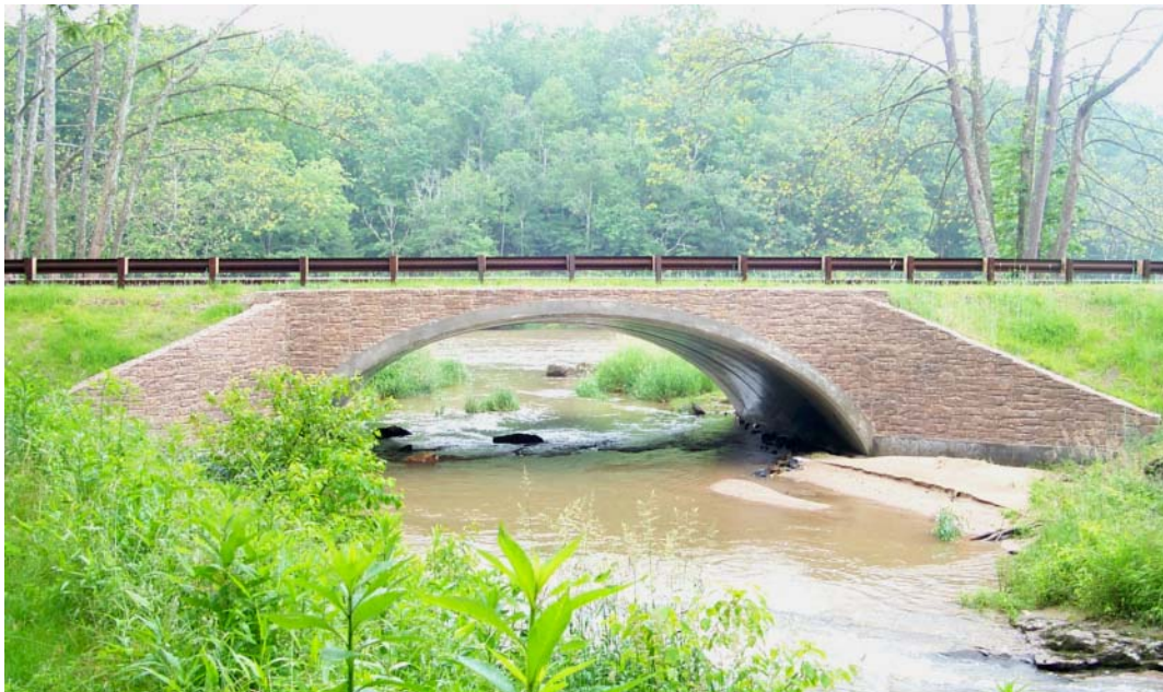
Figure 6: The final appearance was achieved by the use of stained concrete.
