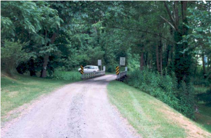
Figure 1: The old Grassy Creek Bridge carried a one-lane gravel road with a clear roadway width of just over 11 feet.
