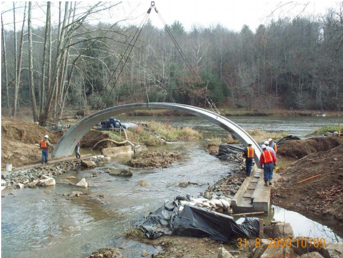
Figure 3: Installation of the first Precast arch segment
