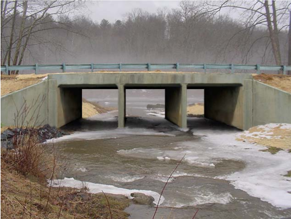
Figure 2: A computer visualization of the project utilizing a triple 12' X 9' RCBC. This option was derided by the community as being visually unappealing.
