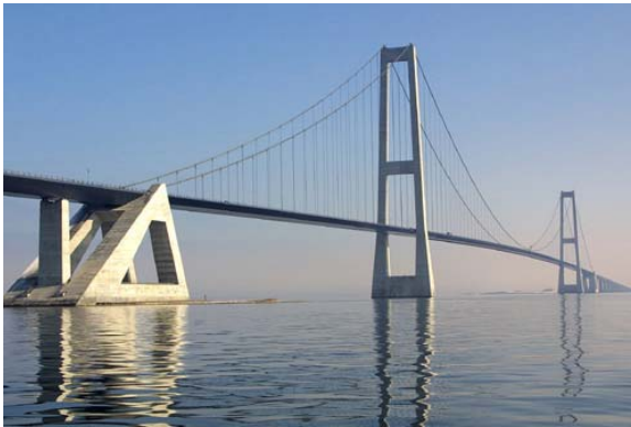
Fig. 2 Great Belt Link (free span of 5328 ft. (1624 m)), Denmark.
