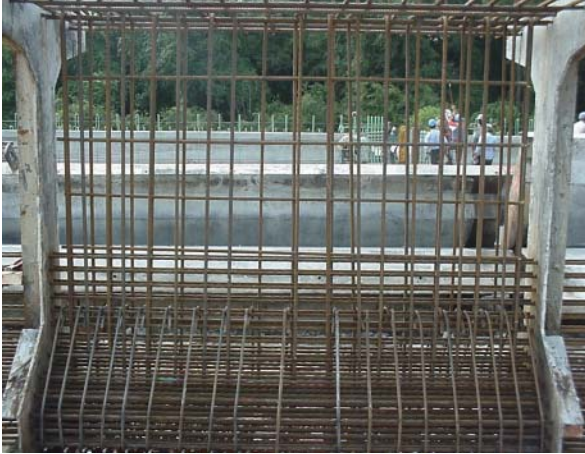
Fig. 1 Beam mock-up section
