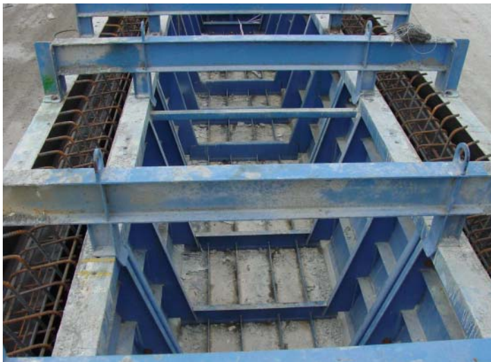
Fig. 10 Formwork for U-beam
