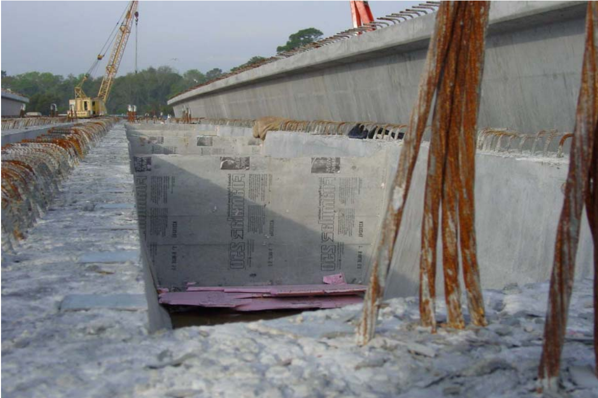
Fig. 12 U-Beams for the SR 9A – I-95 – I-295 projects, inside and outside surface finish
