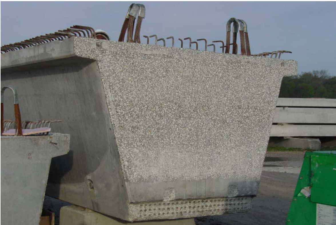
Fig. 13 Exposed header of U-beam shows the uniformity of aggregate distribution
