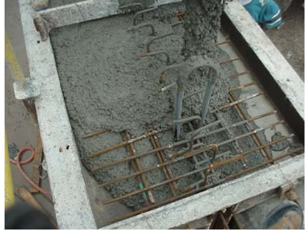
Fig. 2 Casting with flowing concrete
