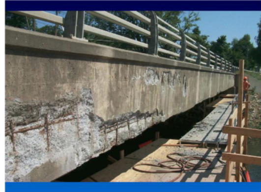
Photo 6 Condition of Precast beams prior to rehabilitation program.
