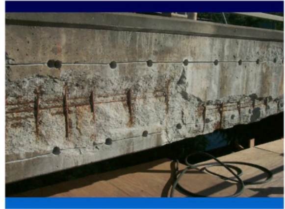
Photo 9 Layout of the galvanic protection system prior to installation.
