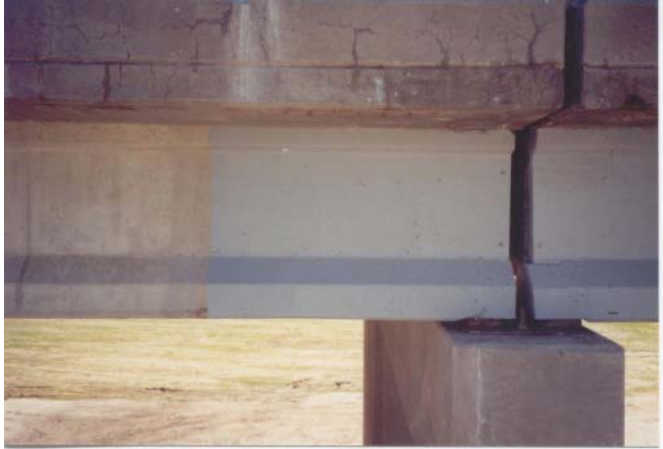
Photo 5 Completed prestressed beam end repair with embedded galvanic protection
