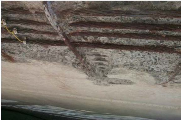
Photo 7 Electrical continuity established between the exposed strands
