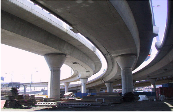
Fig. 5: Curved interchange ramps
