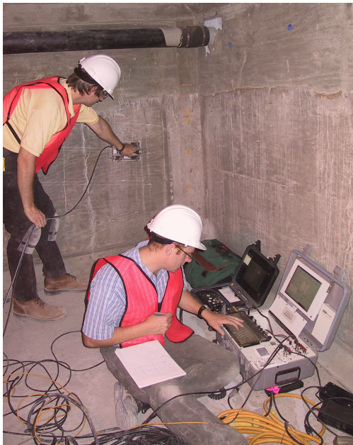
Fig. 17: Echo-impact testing underway.
