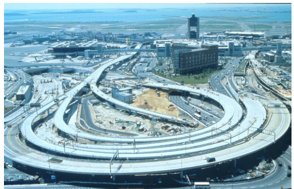
Fig. 4: Logan Airport/I-90 Interchange
