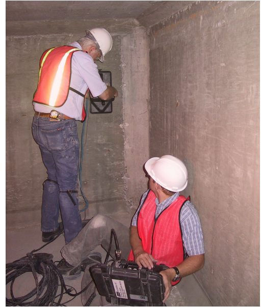
Fig. 16: GPR investigation in progress.
