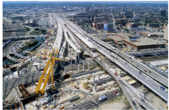
Fig. 2: South Bay Interchange under construction
