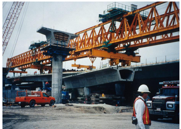
Fig. 3: Cantilever erection using gantry
