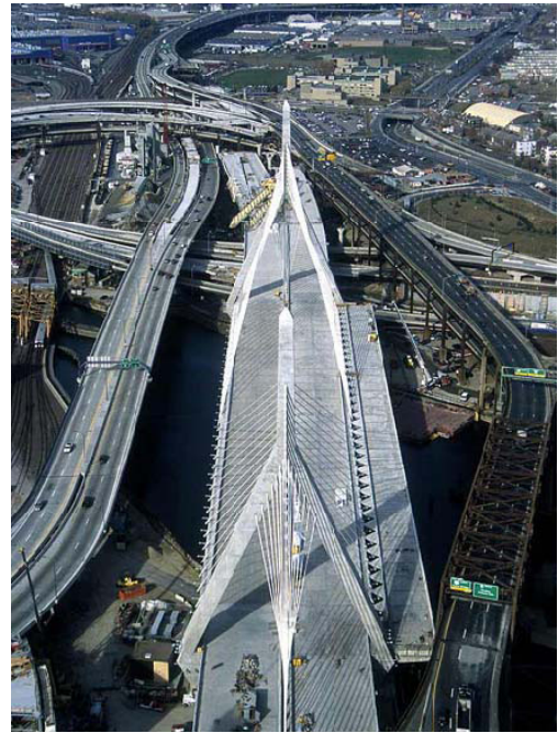
Fig. 9: Stay cable layout on the bridge
