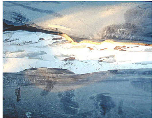
Fig. 5 Strand Corrosion from Cracked PE Duct
