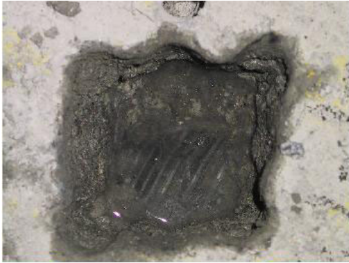
Fig. 1 Drilling to Duct
