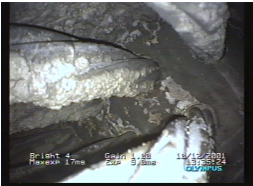
Fig. 10 Void in Top of Duct Existing Construction
