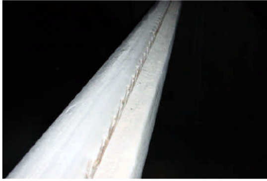
Fig. 13 Bleed Trail in Draped Tendon PE Pipe Removed
