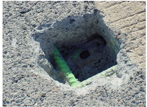
Fig. 2 Removal of Concrete
