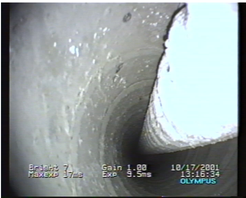
Fig. 10 Void in Top of Duct Existing Construction
