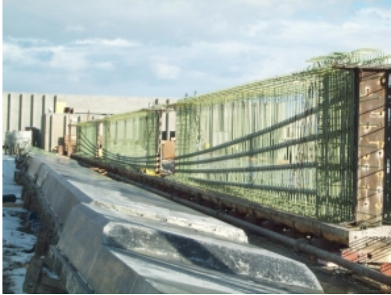
Fig. 1. Casting of Girder A
