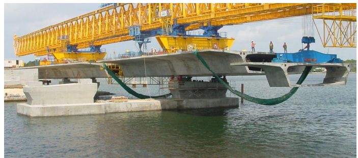
Figure 1 – Combined Waterline Pile Cap
