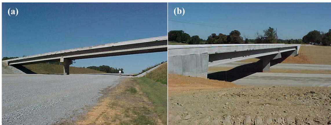
Fig. 1 Tennessee's HPC Showcase Bridges: (a) Porter Road Bridge; (b) Hickman Road Bridge
