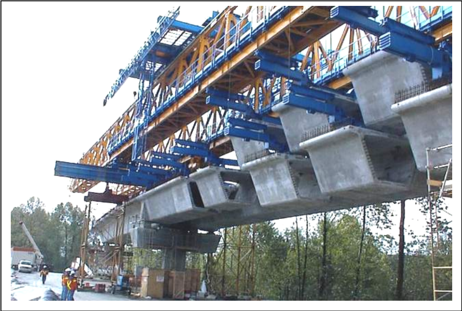
Figure5: Typical Span Erection with “Combi” Truss
