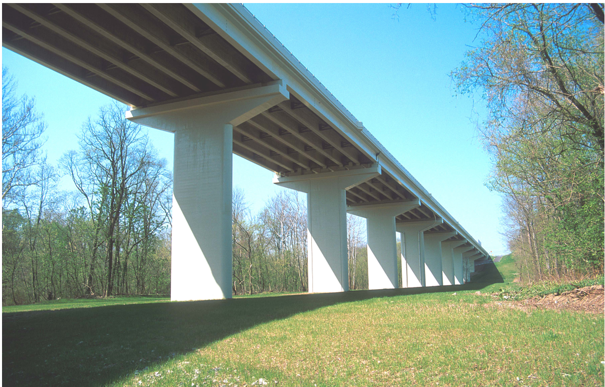
Fig. 9: Lorain Bridge Looking West
