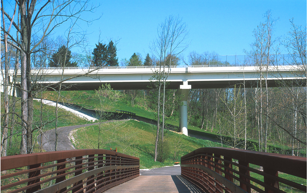
Fig. 15: Spans 1 & 2 as seen from Bike Path
