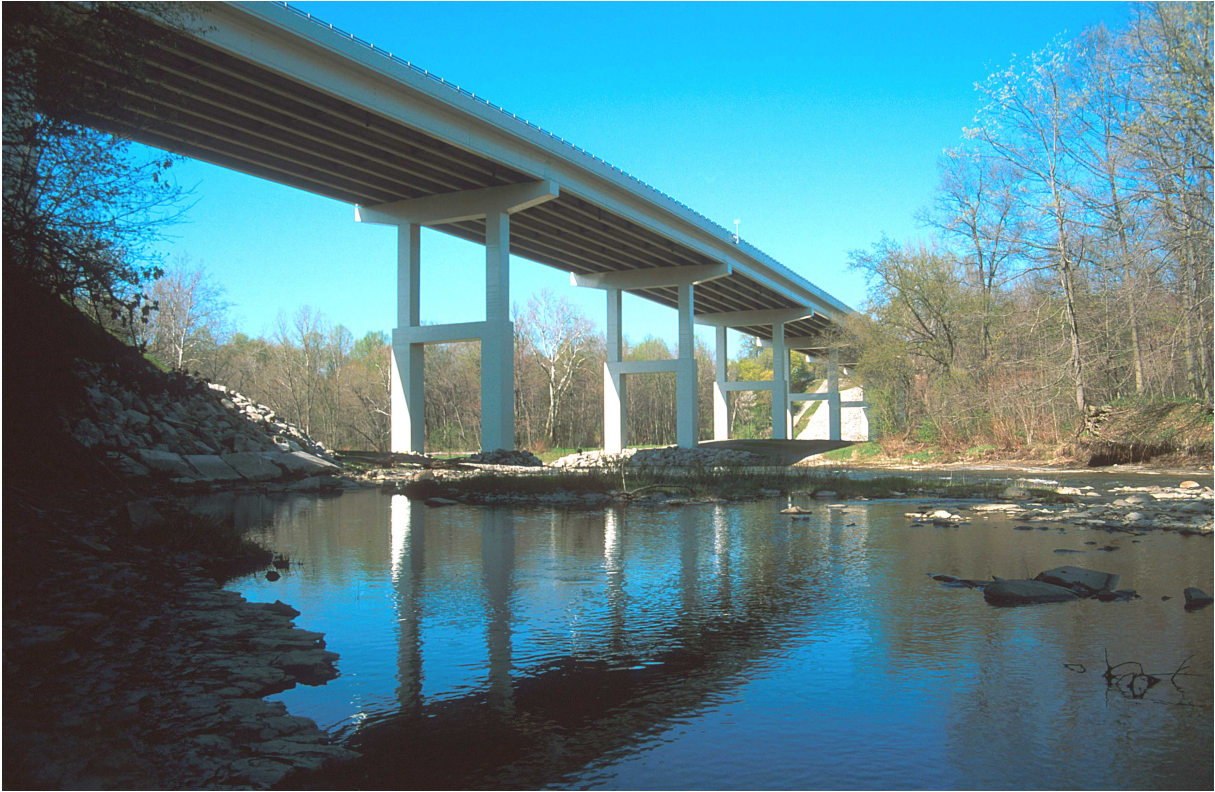
Fig. 1: Ashtabula Bridge Looking East
