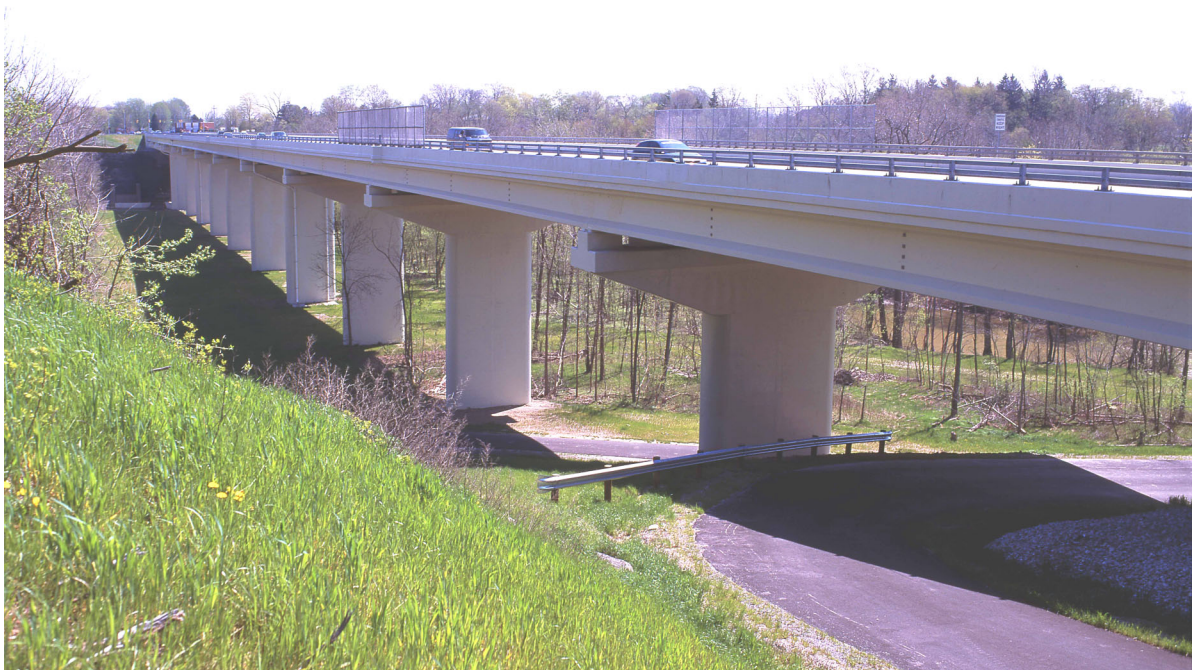
Fig. 14: Lorain Bridge Looking East
