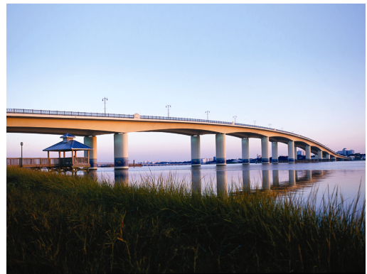
Fig. 3 - The Broadway Bridge features 262’ typical spans as it crosses the Halifax River, which is also the Intracoastal Waterway in this area.
