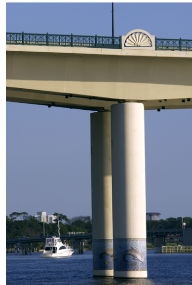
Fig 4. – Ten foot tall mosaics wrap each of the 26 piers on Broadway Bridge.
