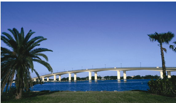
Fig. – The completed Broadway Bridge has become a local landmark and a source of great pride for local residents who participated in the community charettes.
