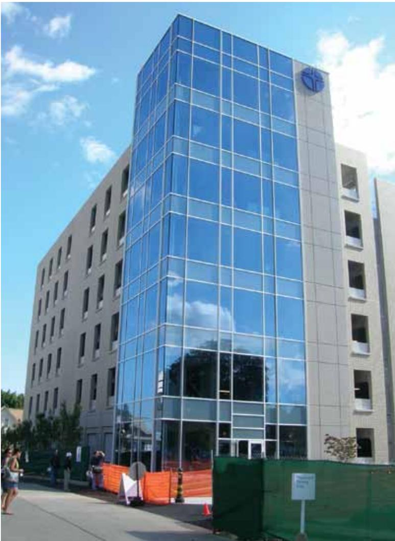
The St. Vincent's Medical Center parking structure in Bridgeport, Conn., met budget, time, and site constraints with precast concrete. Photo © Vince Streano [www.streano-havens.com](http://www.streano-havens.com).
