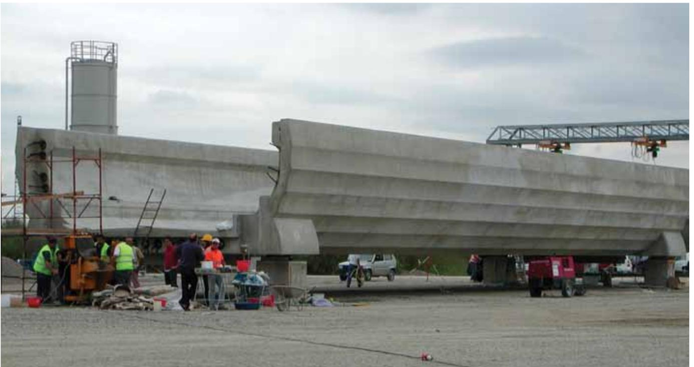
**Figure 6.** Span storage.
