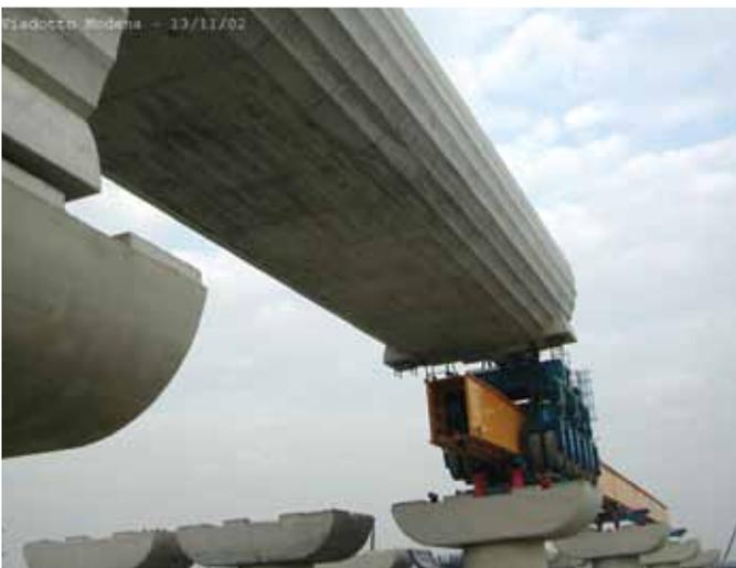
**Figure 10.** Forward launching of the underbridge.
