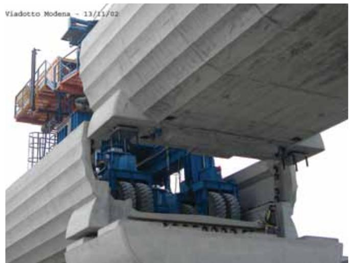
**Figure 11.** Final lowering of the span.
