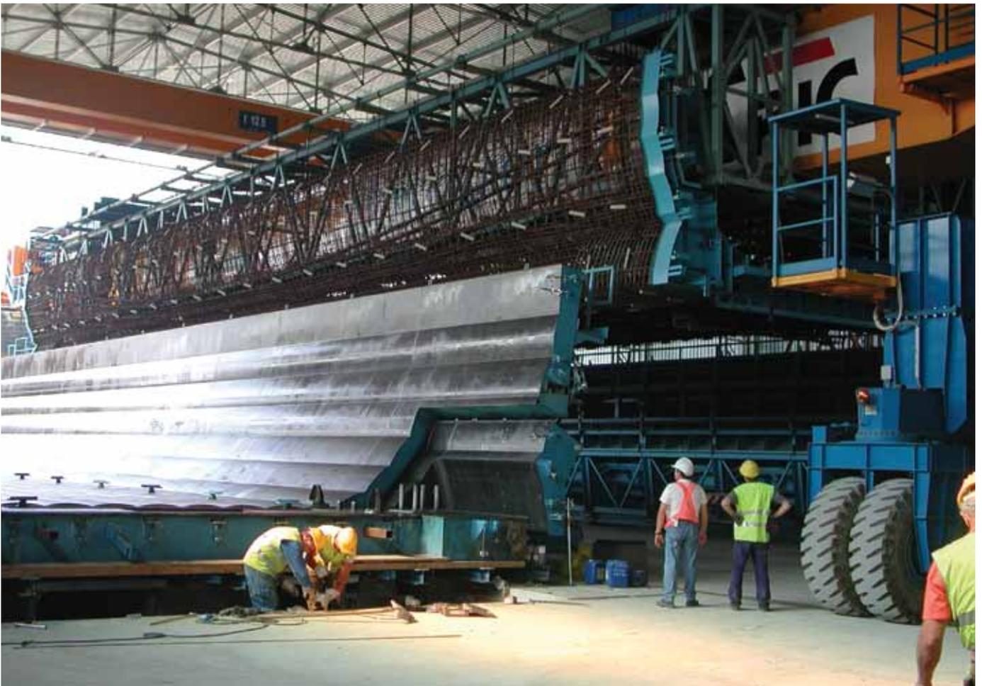
**Figure 2.** Cage delivery to the form.
