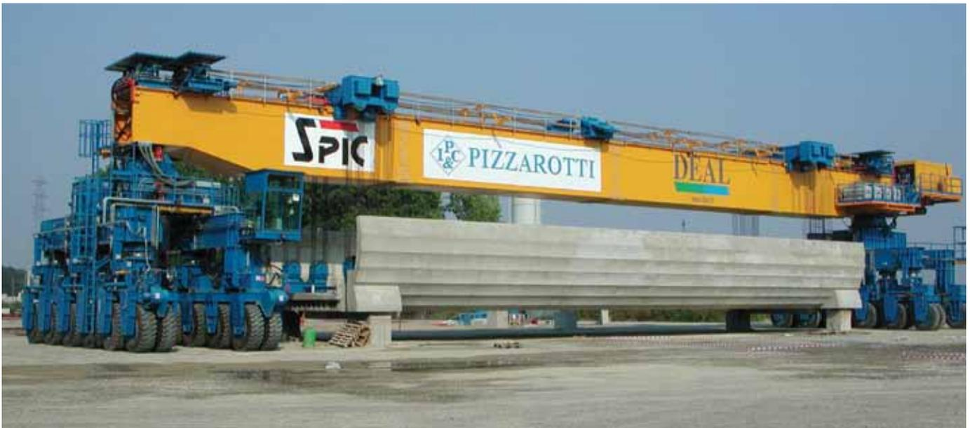
**Figure 7.** Span being lifted from the storage area.
