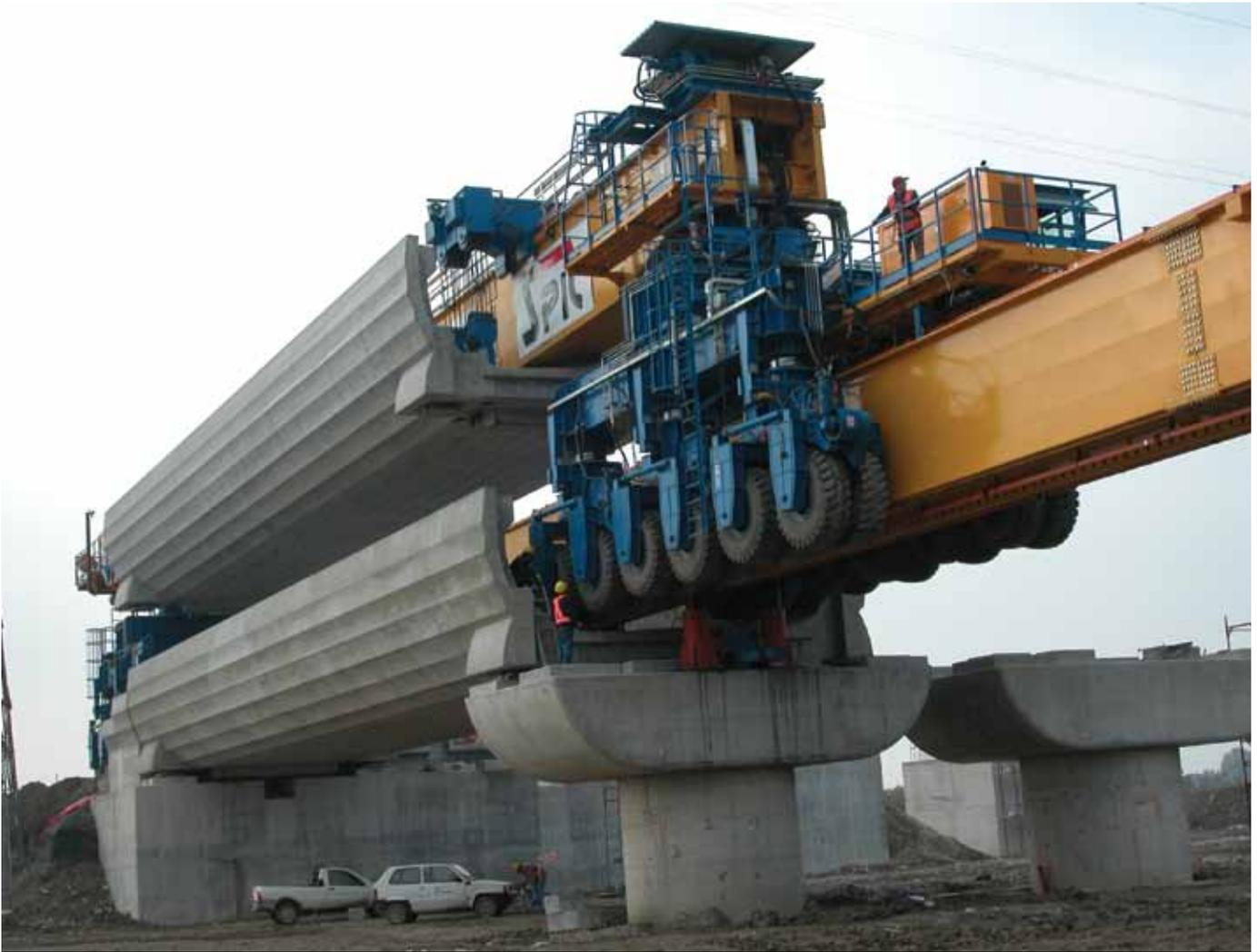
**Figure 9.** Front trolley advancing along the underbridge.
