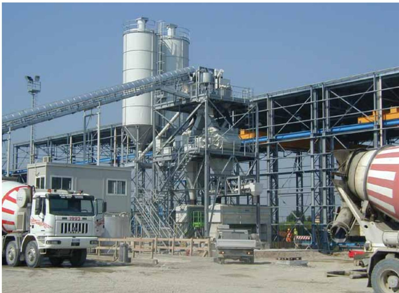
**Figure 4.** Batch plant.
