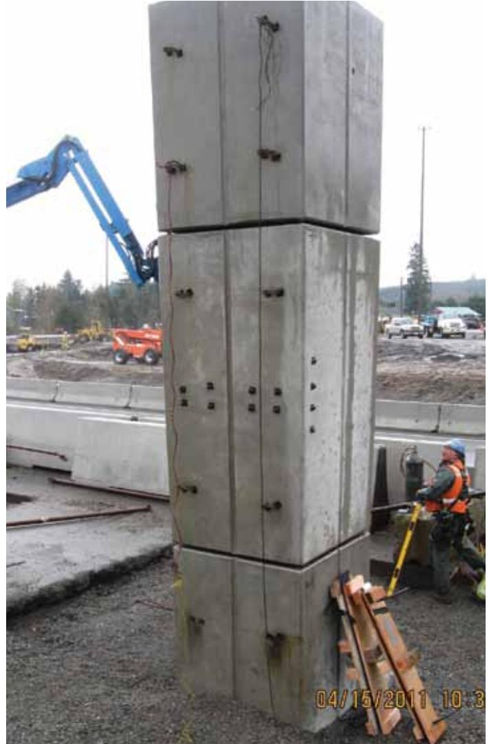
**Figure 14.** Placement of column segment.
