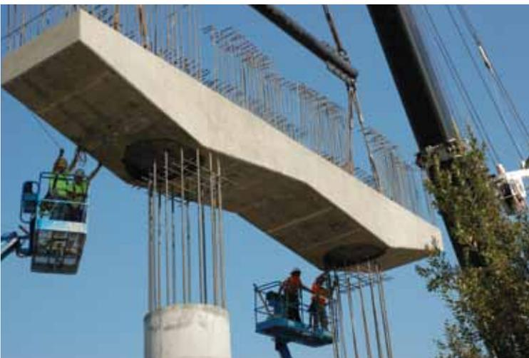
**Figure 4.** Previous use of precast concrete cap beam that used a large number of column bars in a seismic area of Washington State.
