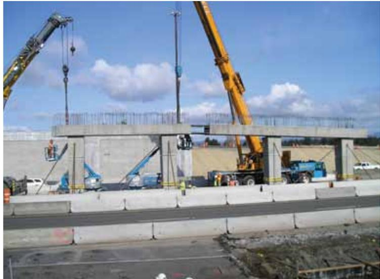
Figure 15. Placement of precast concrete cap beam.
