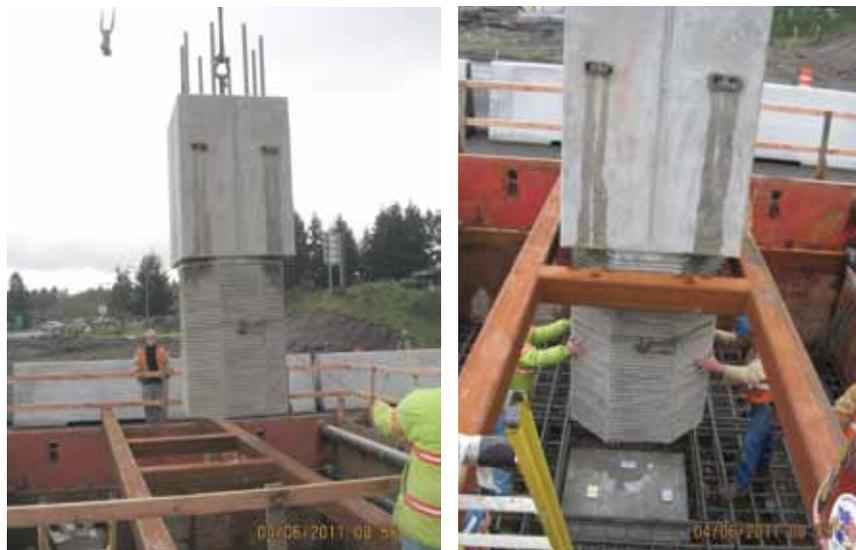
**Figure 13.** Construction sequences for placement of precast concrete column segment into footing.
