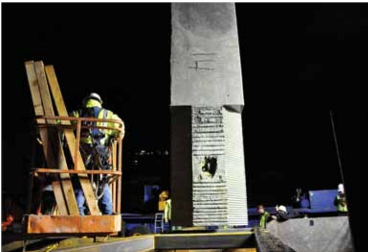
**Figure 3.** Socket connection concept.
