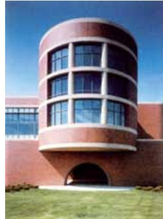
**Figure 1** Radial brick was cast into radiused precast concrete panels for the S.C. Johnson Worldwide Professional Headquarters in Mt. Pleasant, Wis., to create the smooth flow around corners. (Architects Zimmerman Design Group and Hellmuth, Obata & Kassabaum, Inc.)
