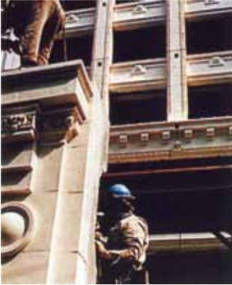
**Figure 6** Built in 1906, the architectural landmark 88 Kearney St. in San Francisco had its terra cotta removed and reassembled on precast panels for an all-new structure of taller height. (Architect Skidmore Owings & Merrill)
