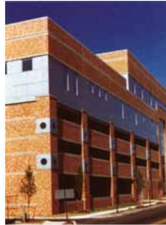
**Figure 11** The perimeter columns and wall components of the St. Peter's Ambulatory Surgery and Parking Structure in New Brunswick, N.J., were cast with dovetail slots to facilitate quick installation of full brick in the precaster's yard. (Courtesy Robert Mueller Architectural Photography)
