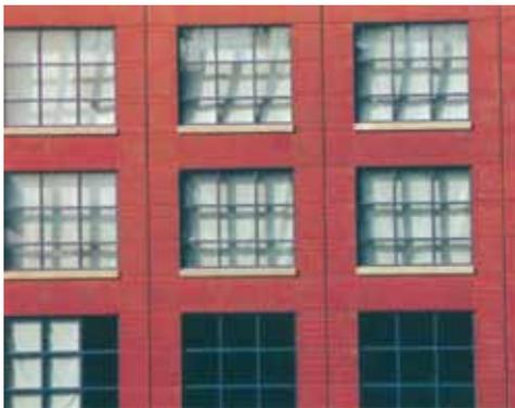
At the USTA National Tennis Center, the brick was tuck pointed after being cast into panels. The weight of the precast concrete panels is carried on the foundations of the building.
