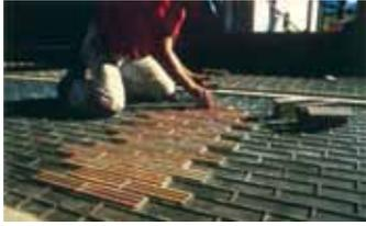
**Figure 8** Thin brick is shown being placed in an elastomeric form liner.
