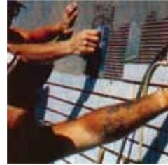
**Figure 10** Glazed thin bricks are tapped unto mortar using a rubber mallet.
