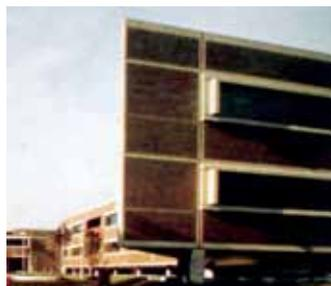
**Figure 5** Spandrels and wall panels on the Sylvan Corporate Center in Englewood Cliffs, N.J., have integrally cast 8-inch-square brick-colored tiles with pigmented mortar. (Architect Herbert Beckhard Frank Ricklan & Associates)
