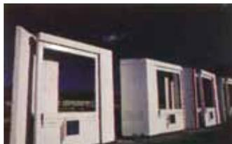
**Figure 4** These panels have 6-inch-square glazed white ceramic tiles and some additional 10-inch-square accenting blue tiles.
