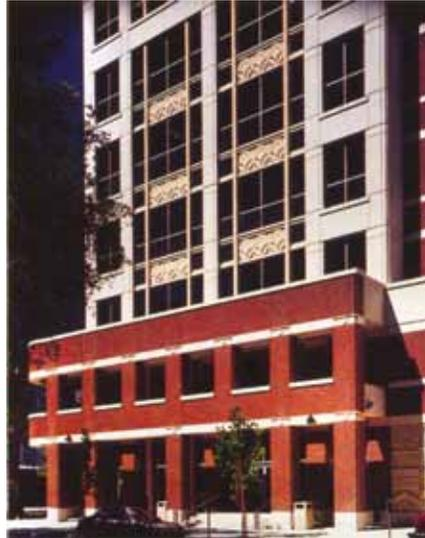
**Figure 7** One-inch-thick brick cladding on 5-inch-thick concrete panels was used on the first three floors of the Sacramento County System and Data Processing Building in Sacramento, Calif. Terra cotta medallions were placed on spandrels and column covers (Architect Ehrlich-Rominger)
