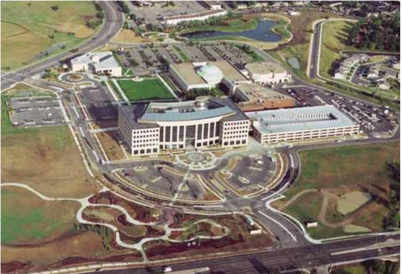
Fig. 1. Looking westward, an aerial photograph captures the visual impact of the clean, classic design lines of the east elevation of the new City of Aurora Municipal Building. The stately structure works in harmony with landscaping and existing city buildings. [Photography courtesy of Aerial Arts]
