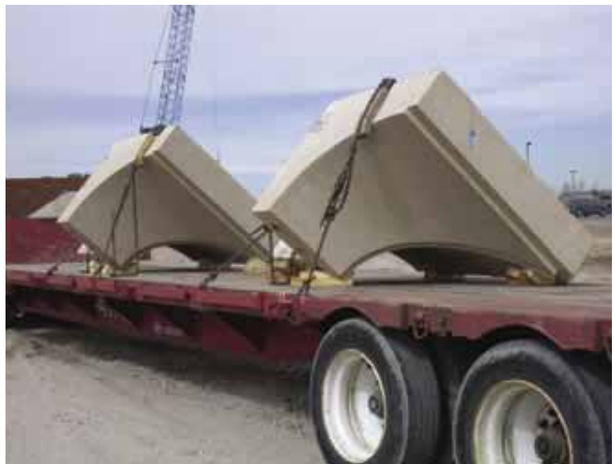
Fig. 16. Trailer bed transport of two curved precast concrete parapet pieces. Production of these projecting parapets required high skill and tight tolerances.
