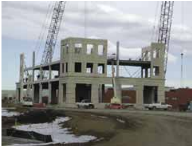
Fig. 19. A “tower” construction method facilitated erection in several locations at once.
