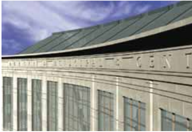
Fig. 18. Rooftop loads were reduced by using a lightweight metal enclosure around the mechanical penthouse.
