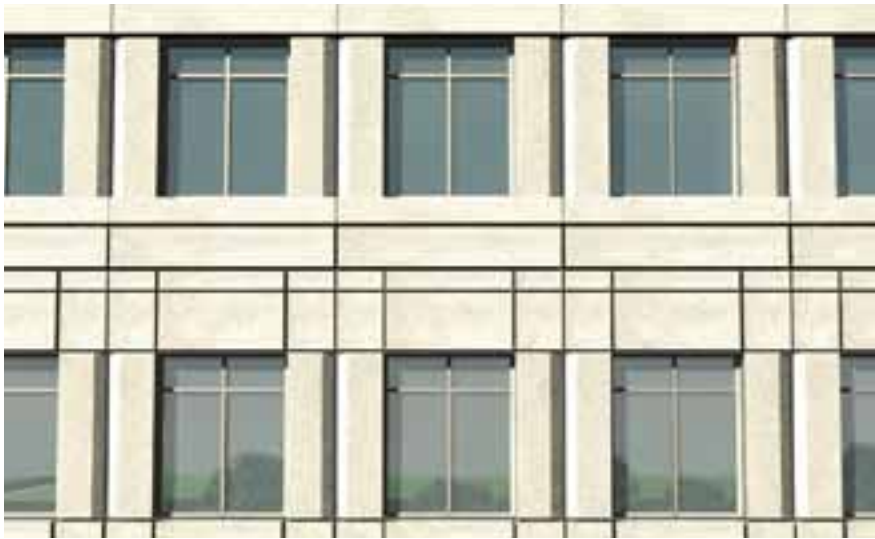
Fig. 6. Punched window detailing in wall panels is testimony to the design versatility and inherent attractiveness of architectural precast concrete.
