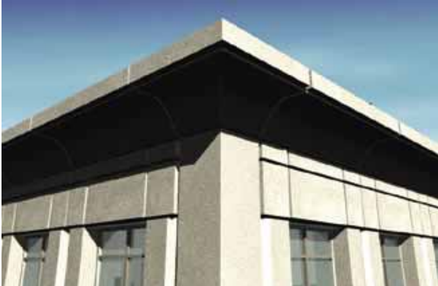
Fig. 13. View of corner cornice detail.
