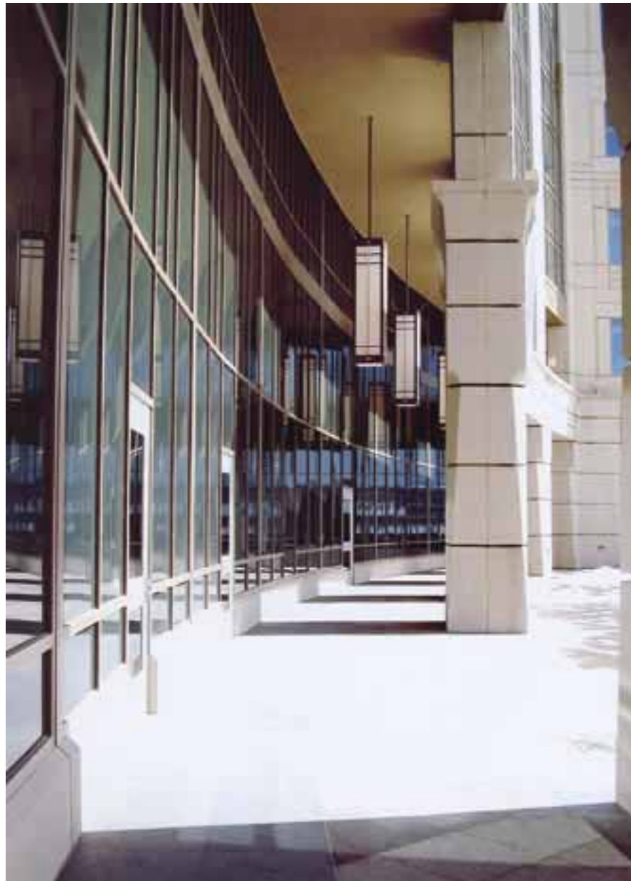
Fig. 12. An elegant loggia with free-standing precast concrete columns greets visitors to the complex.
