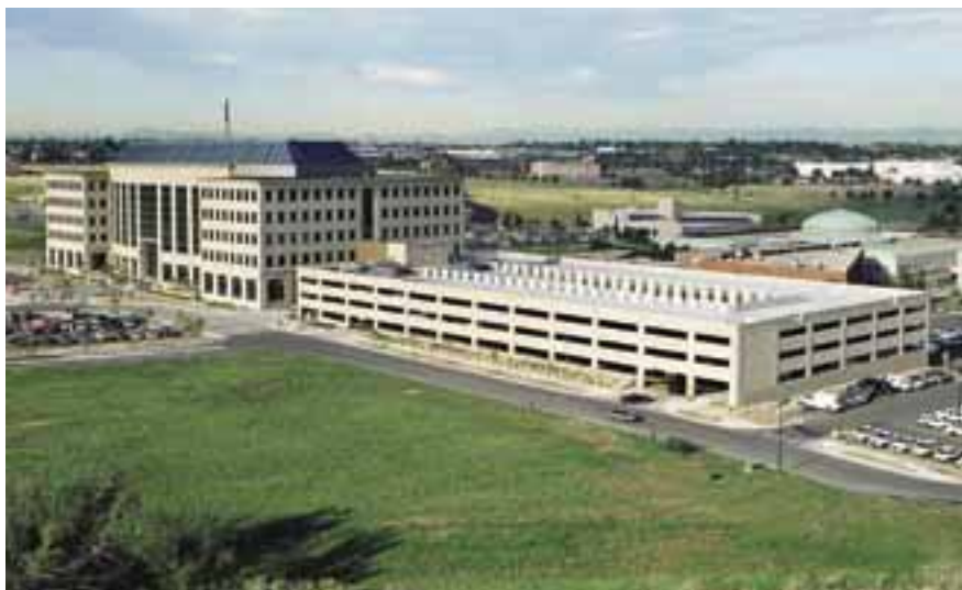
Fig. 8. The neoclassical style continuity of both structures is apparent in this aerial photo of AMC from the vantage of the parking structure. [Photography courtesy of Aerial Arts]
