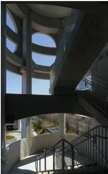
Design features enhance the exterior appearance of the stair tower, which, from the inside, is appealing in its openness. Photos: ©EricTaylorPhoto.com
