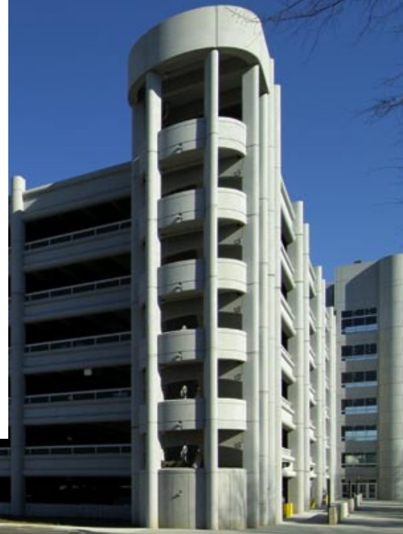
The total-precast parking structure at Shady Grove station on Washington, D.C.'s Metro red line has visual appeal as well as functionality. The stair tower at left adjoins an elevator tower. Photos: ©EricTaylorPhoto.com
