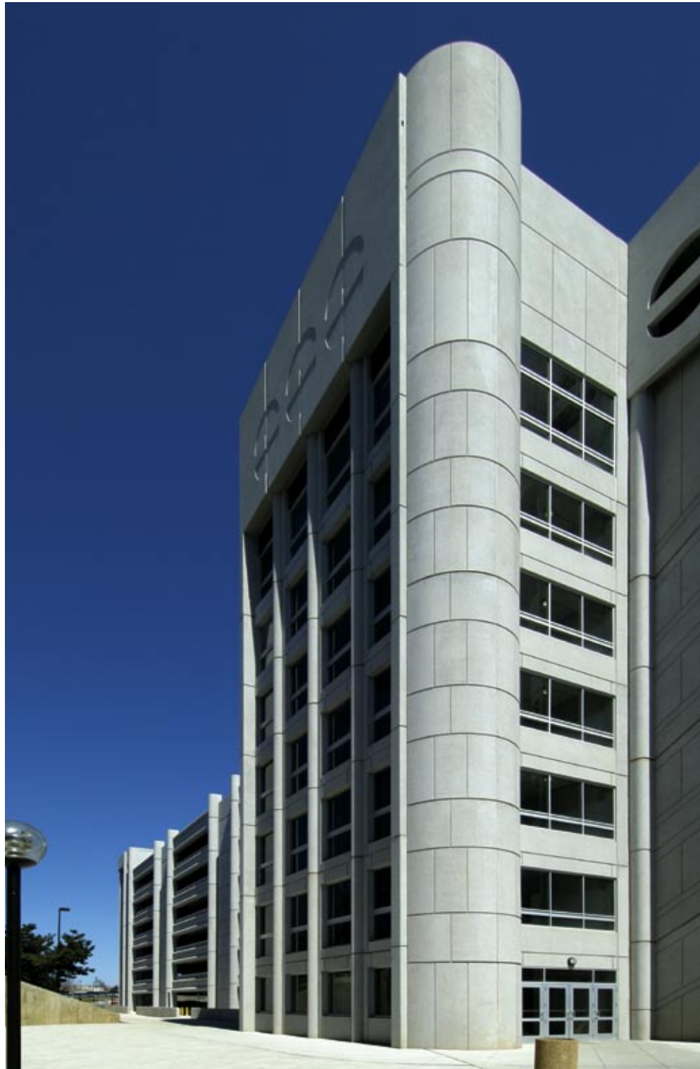
The elevator tower is enclosed in glass, one of the few non-precast components in the garage. Photos: ©EricTaylorPhoto.com
