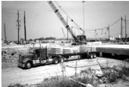
Figure 16.2.4.5-1 SIP Deck Panels being Delivered to Bridge Site
