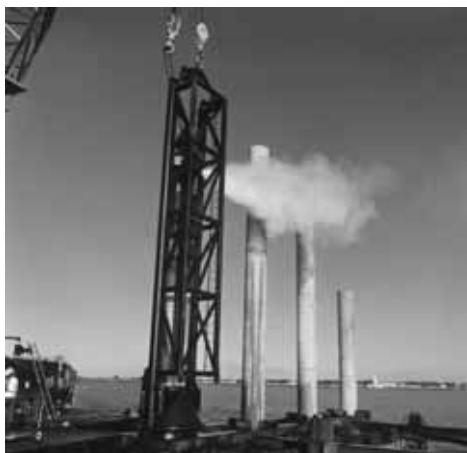
Figure 16.4.4-1 Driving Cylinder Piles
