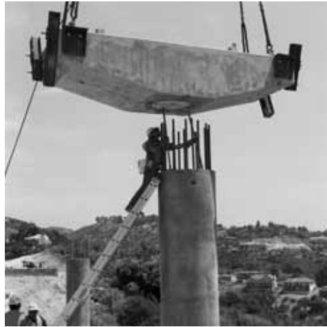
Figure 16.6.2-1 Erection of Precast Cap over Column Dowels
