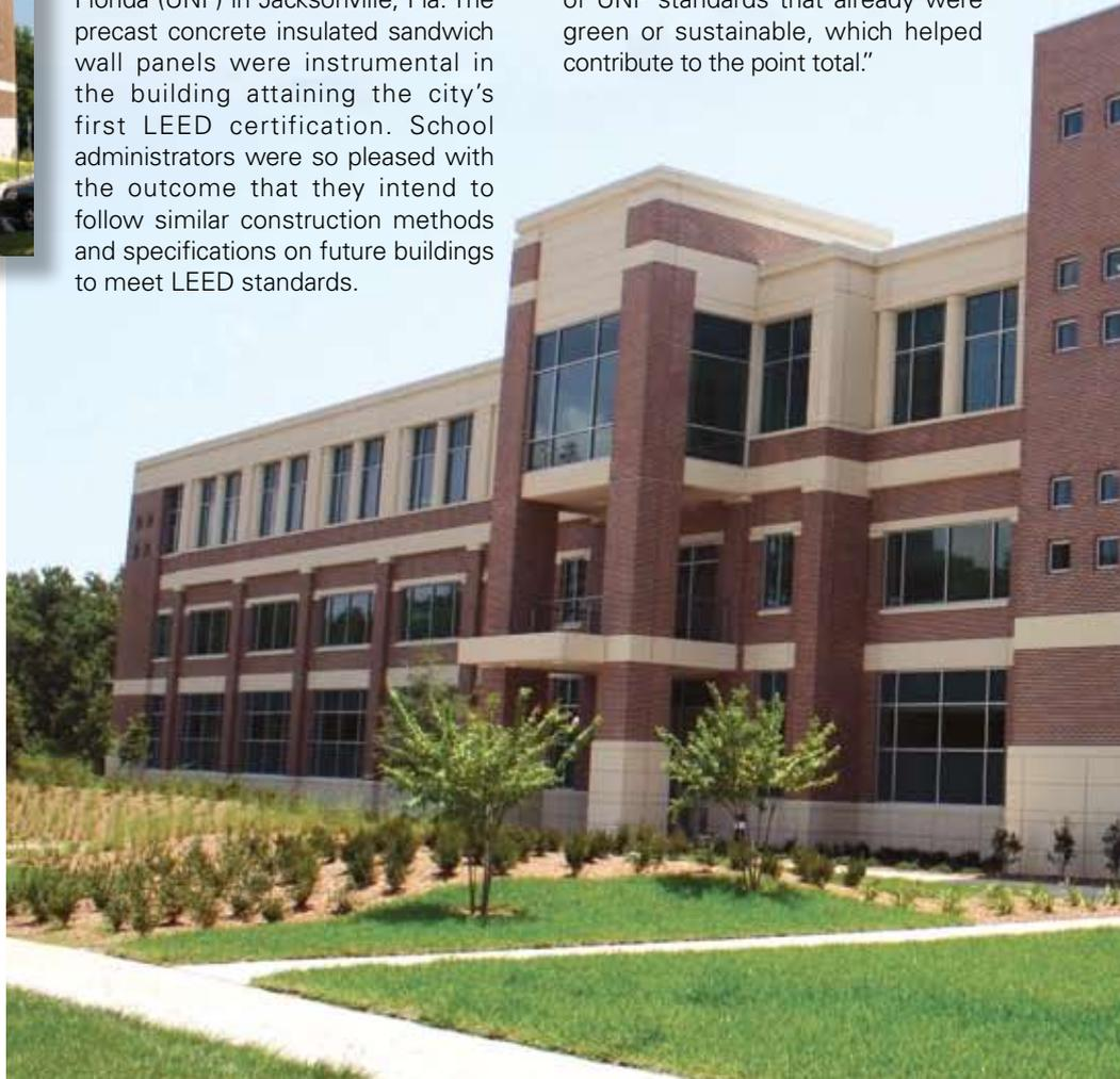
Jacksonville, Fla., university uses thin-brick systems and thermal analysis along with precast concrete insulated wall panels to achieve certification
