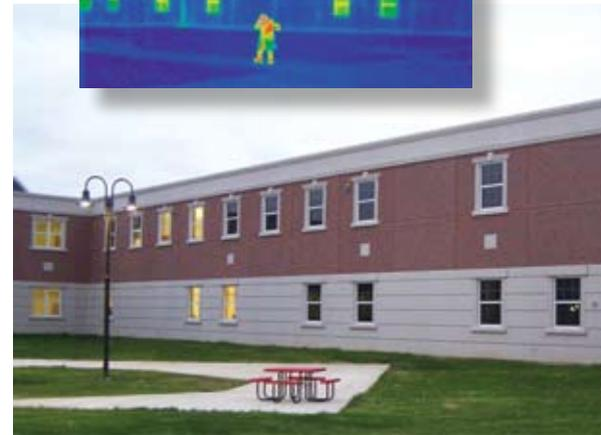
Thermal-imaging studies use infrared rays to detect the amount of heat energy in a location. These “after” images with precast concrete panels in place on a high-school project, show the low-heat blues and greens that are desired rather than the red/orange “hot spots” that indicate energy loss.
