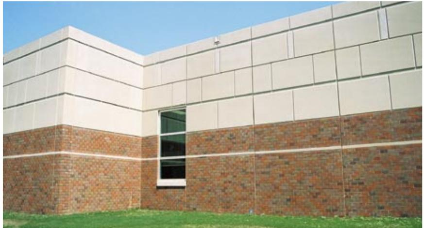
Panels at both schools featured thin brick on the lower portions. The brick was cast into the panels at Rinker's plant. The upper portions simulate limestone.
