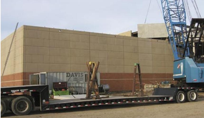
A single crane was needed for erection of both schools. Here, it swings panels into place at Lincoln Southwest High School after plucking them from Rinker's delivery truck.
