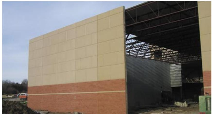
Panels averaged 30 feet high by 10 feet wide and were erected in sequence. Some panels, where greater clearance was needed (such as in the auditorium) were nearly 60 feet high. This shows an early phase of the construction at Lincoln Southwest.
