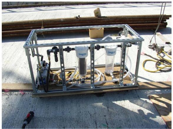
Fig 6 Vacuum pump and protective filters- Benicia-Martinez Bridge, CA
