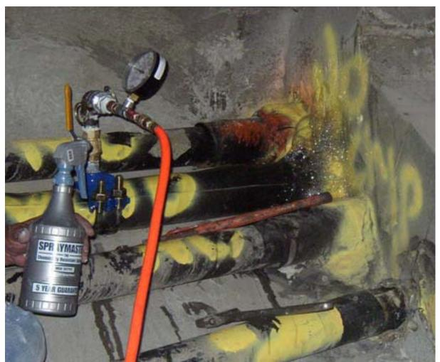
Fig 10. Pressurized Duct with Soapy Water Identifying a Leak- Sunshine Skyway Bridge, Tampa, FL
