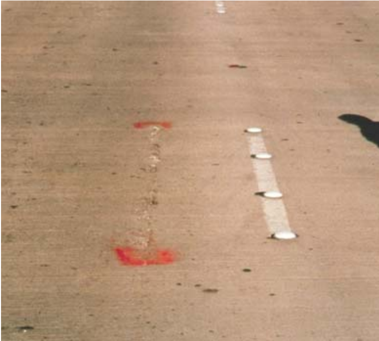
Fig. 9 Large Longitudinal Crack at Panel Edge
