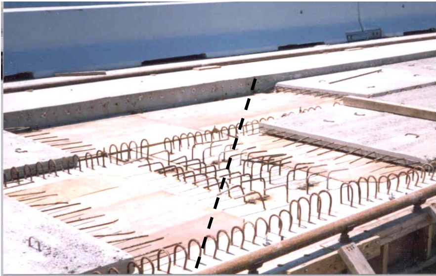
Fig. 3 Staggered Panels on 45° Skew. Note Extension of Reinforcing Steel From Panels; Dashed line indicates centerline of bent
