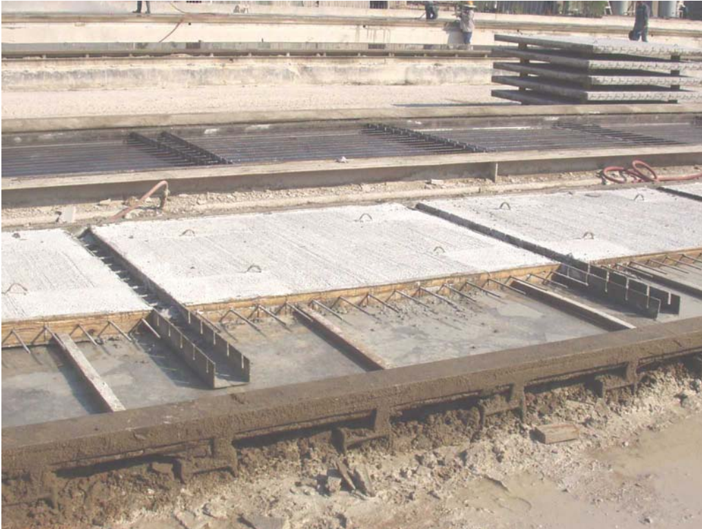
Fig. 6 Forming of End Panel Showing Gap in Forms and #3 Reinforcing Steel
