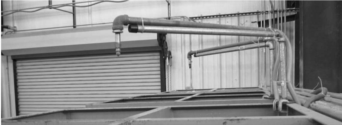
Figure 2. Misting Device Installed Over Aggregate Hoppers
